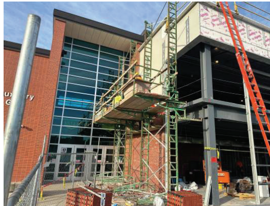
East Wall Brick Install
