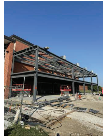
Columns and Beams Set
