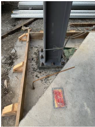
Grout Column Base Plates
