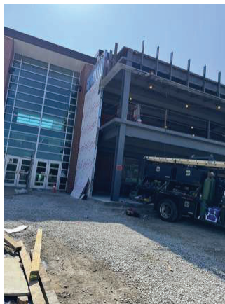
Exterior Framing and Sheathing
