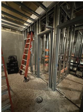
Restroom Wall Framing
