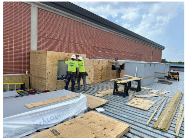
Roof Dog House Wood Blocking
