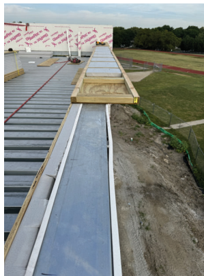
Roof Parapet Blocking
