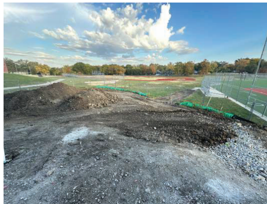
Grading For Sidewalk
