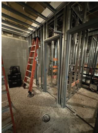
Restroom Wall Framing
