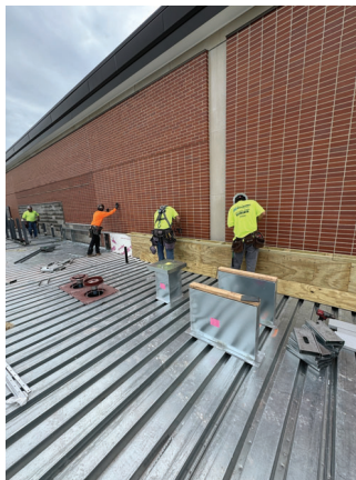
Roof Blocking and Sheathing
