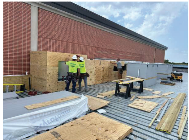
Roof Dog House Wood Blocking
