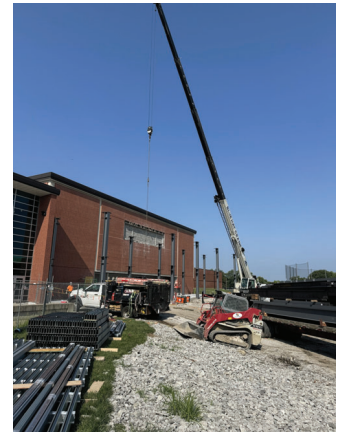
Building Addition Set Columns
