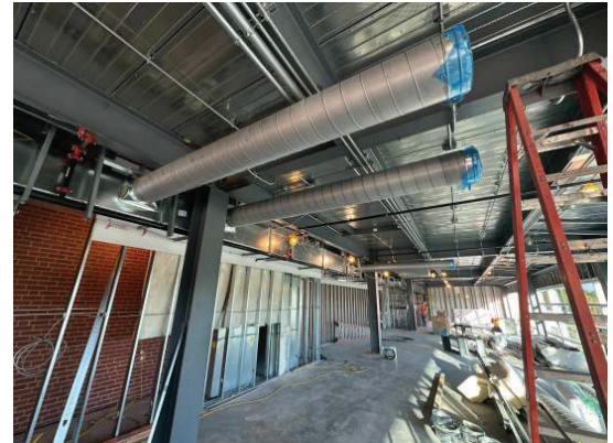
Main Level Ductwork
