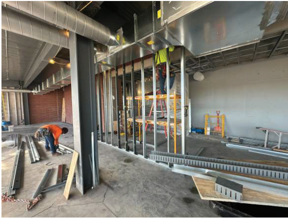
Interior Wall Framing
