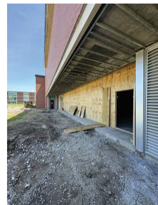
Exterior Demo and Temp Wall For Weight Room
