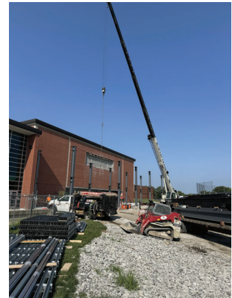
Building Addition Set Columns
