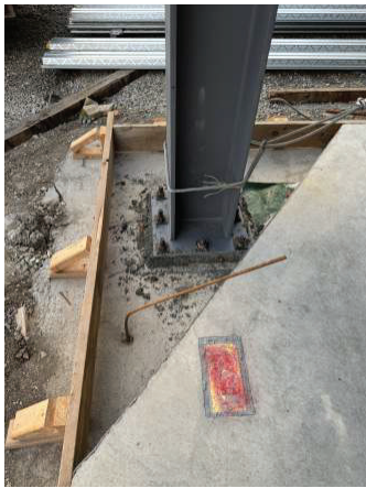
Grout Column Base Plates
