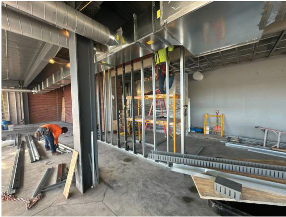
Interior Wall Framing
