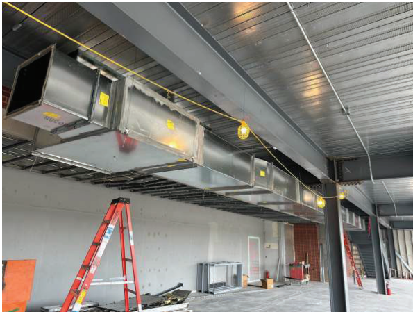
Lower Level Duct Work
