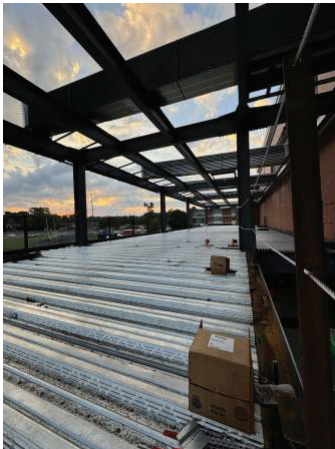
2nd Level Steel Deck
