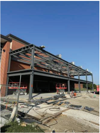
Columns and Beams Set
