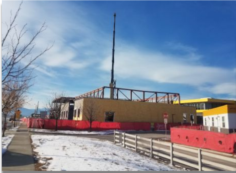
Above: East wall of Gym Addition
