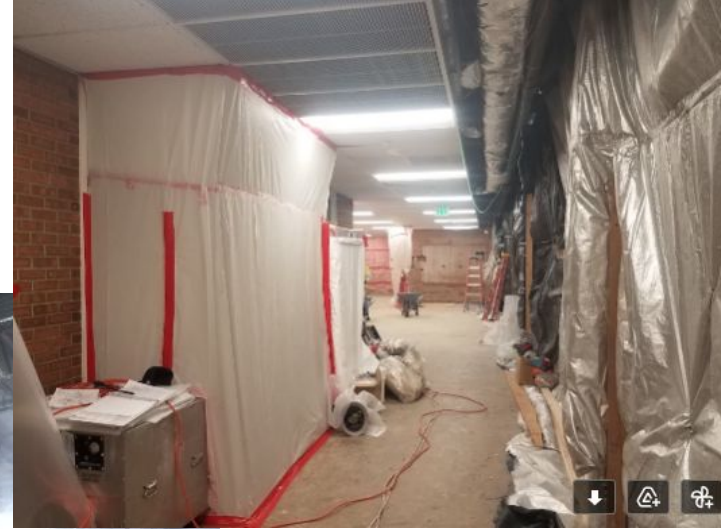
Above: Abatement containment set up for bathroom demolition
