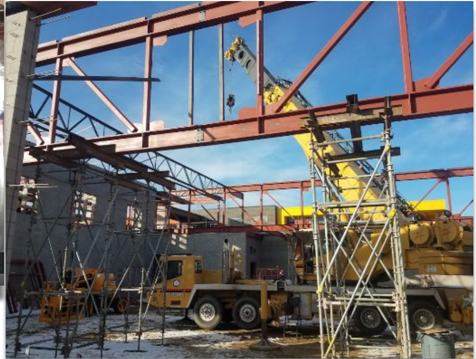
Below: Gym trusses set and ready for joists
