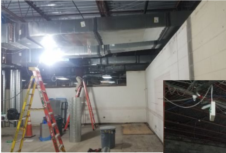
Above: Ductwork for HVAC system
