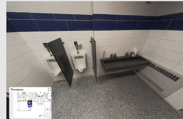
Thompson K-8 - Boys Toilet Room
