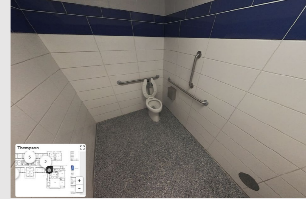
Thompson K-8 - Individual Toilet Room
