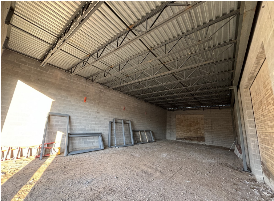
GYM ADDITION STEEL/DECKING COMPLETE
