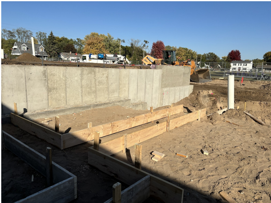
FORM FOOTINGS FOR TECH ED ADDITION
