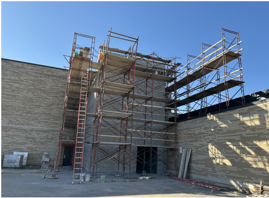
ELEVATOR ADDITION MASONRY
