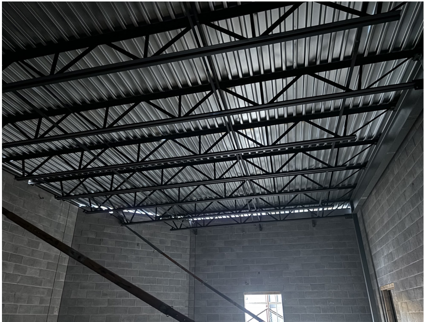
GYM ADDITION STEEL/DECKING COMPLETE
