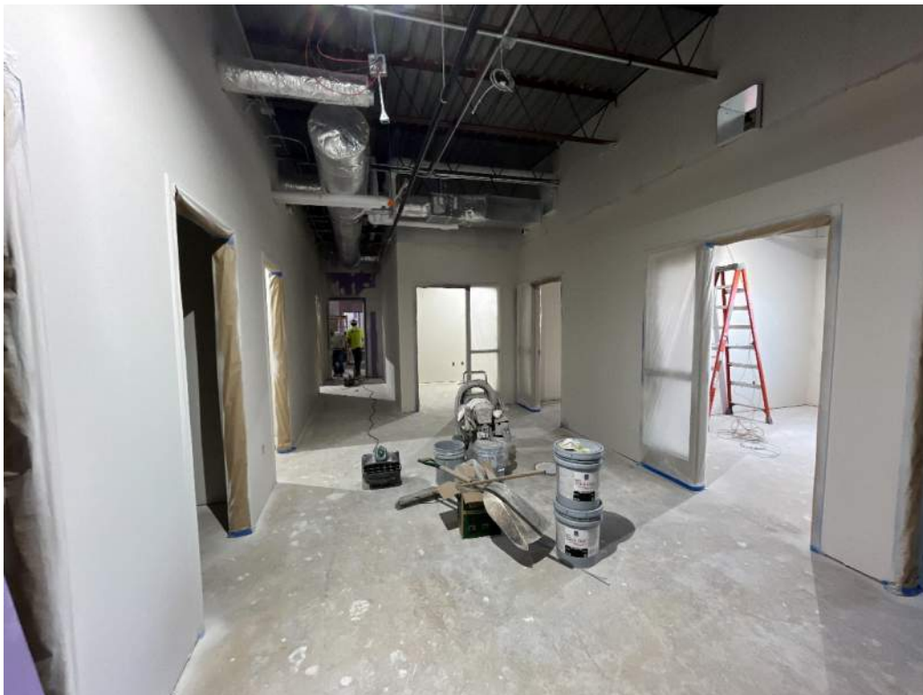
Segment D – School District Admin Area Interior Painting In-Progress
