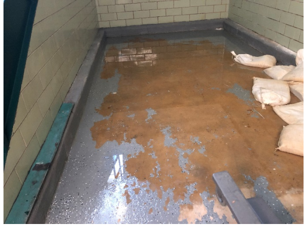
Francis C Hammond, Stairwell View of Floor
