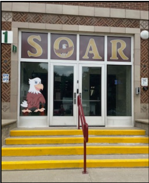
Safety & security additions at entrance
