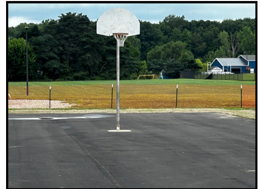
New basketball court surfacing on our playground!
