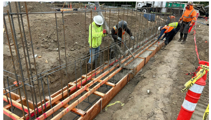
Footing Concrete Placement
