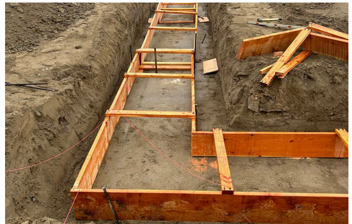
Foot Formwork
