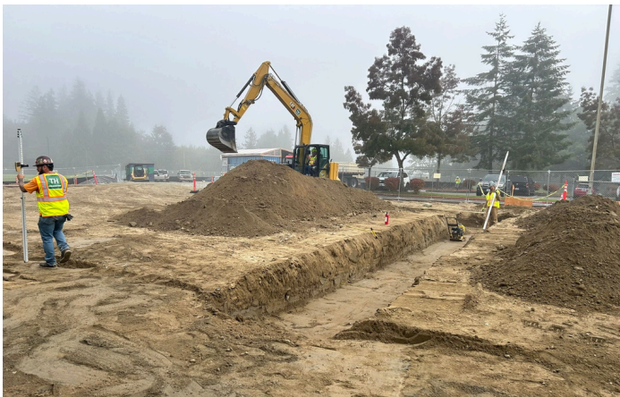
Excavating for Footings
