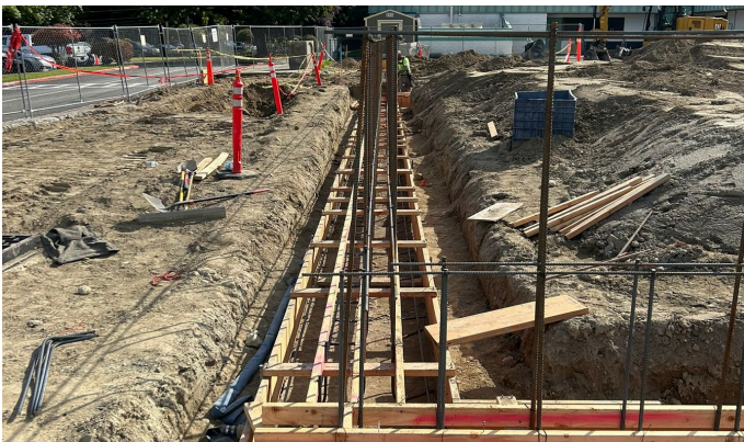
Footing Formwork with Steel Reinforcement
