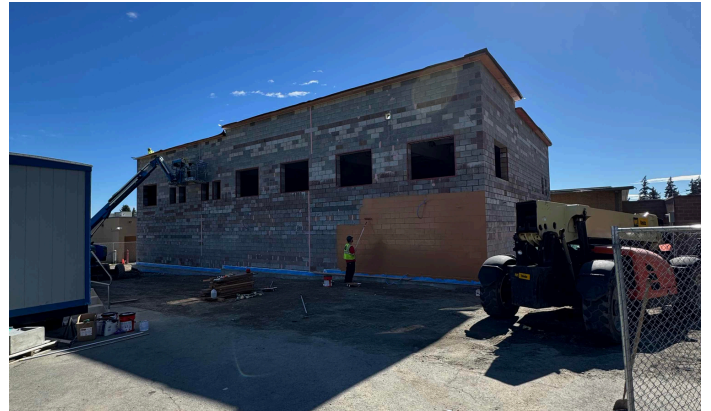
September construction progress
