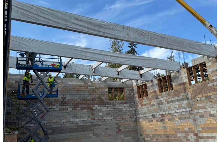
Beam installation
