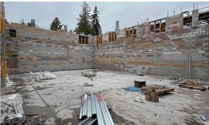
Concrete Masonry Unit Installation
