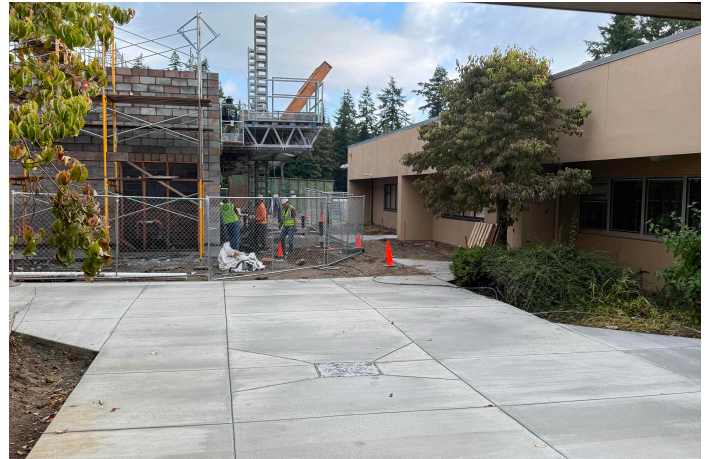
Concrete Walkways Poured
