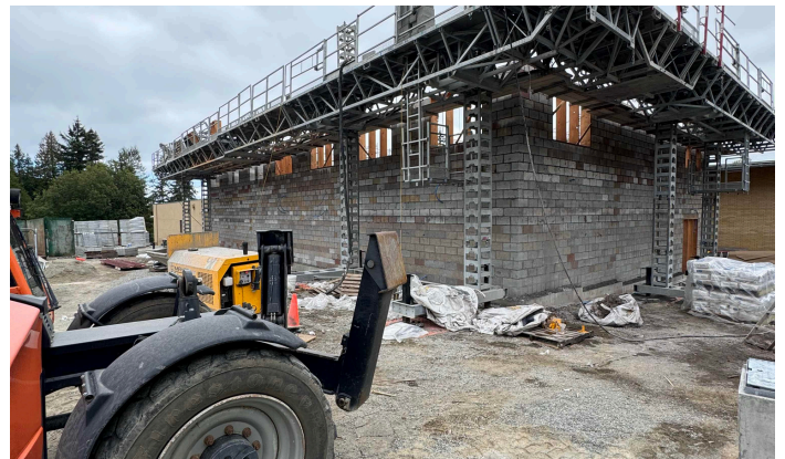
August Construction Progress
