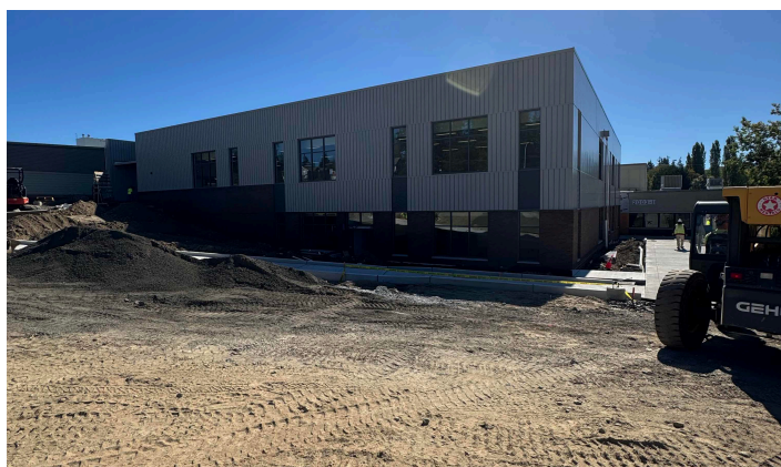
September construction progress
