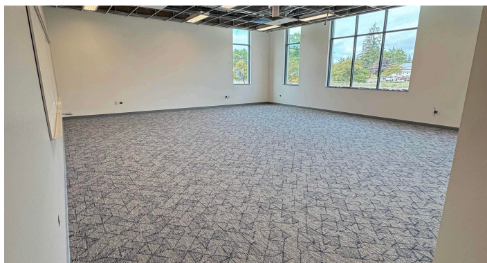
Carpet tile installed
