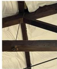
85 year old roof truss in main gym at Mile High Middle School, recently cracked in half. Repairs coming soon!
