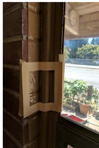
72417-POD-RM04: POD room 4 on window frame.
