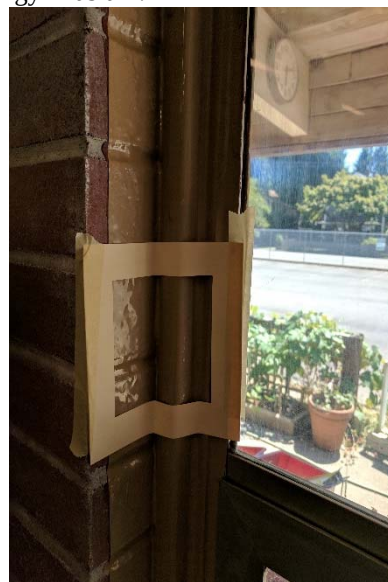
72417-POD-RM14: POD – room 14 on window frame.
