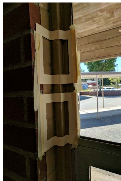
72417-POD-RM20B: POD room 20 on window frame.
