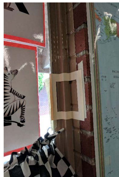
72417-POD-RM17: POD room 17 on window frame.
