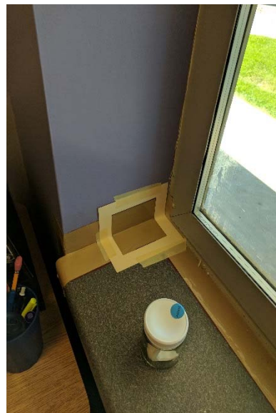
72417-ADM-SEoffice – Admin southeast office window frame.
