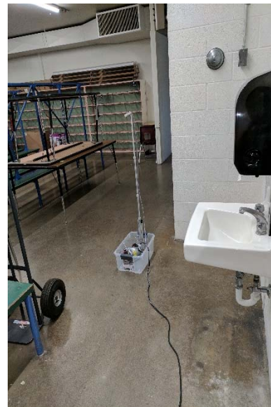
72517-GYM-Girls Lockers: Gymnasium Building girl's lockers.
