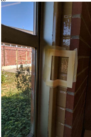
72417-ANX-RMF: Annex room F on window frame.
