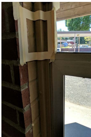
72417-POD-RM20A: POD room 20 on window frame.
