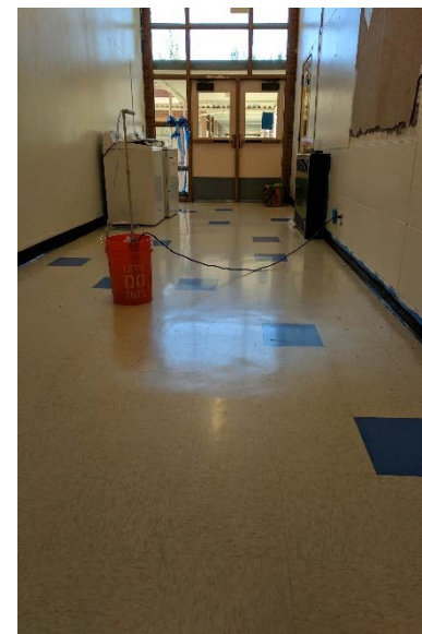
72517-ANX-Ehallway: Annex east hallway.
