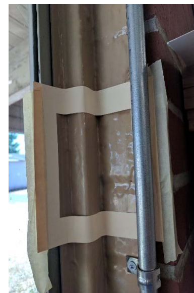
72417-POD-RM11 – POD room 11 on window frame.
