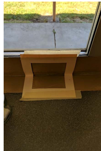
72417-ADM-Woffice: Admin west office window frame.
