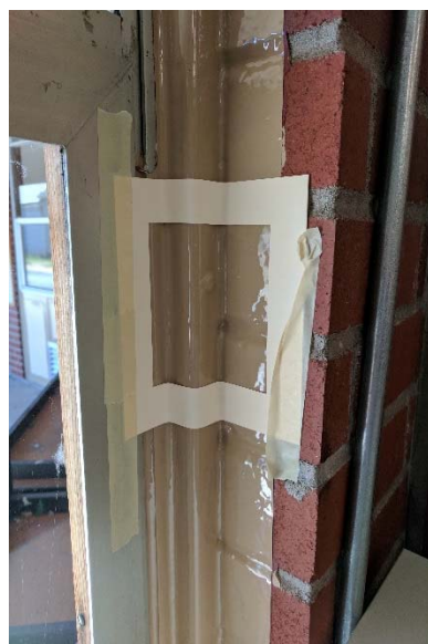
72417-POD-RM08: POD room 8 on window frame.
