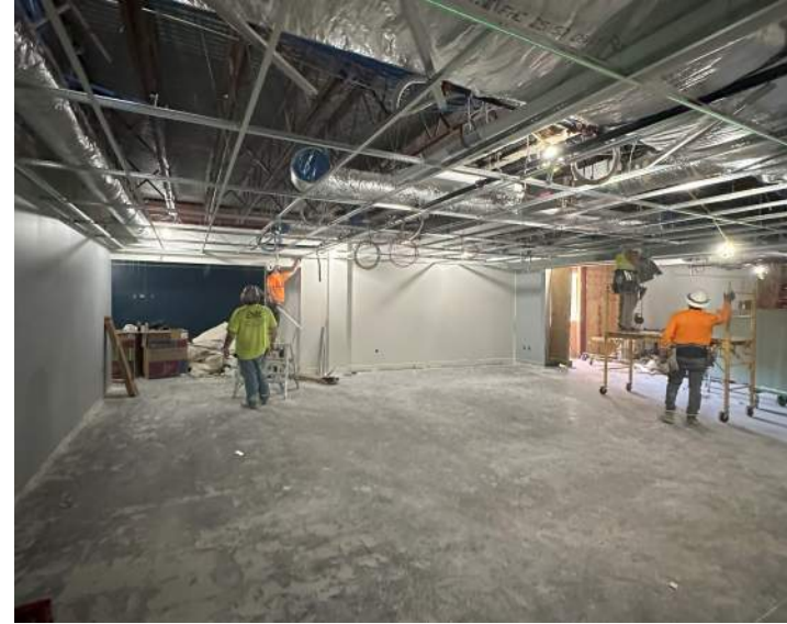
1964 (Area A) Progress
