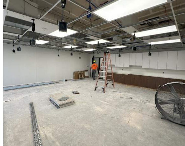
Progress 100's Wing
