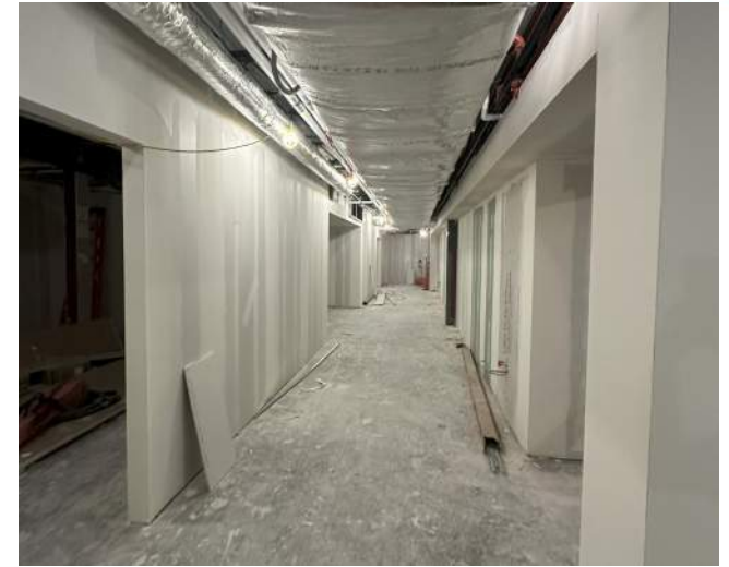
1964 (Area A) Progress
