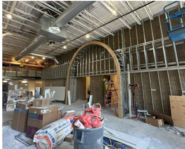
1964 (Area A) Progress
