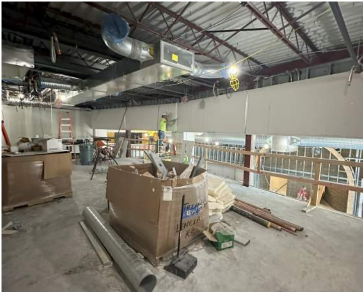
1964 (Area A) Progress
