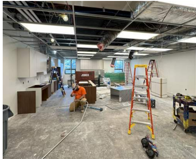
Progress 100's Wing
