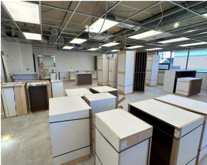
Progress 100's Wing
