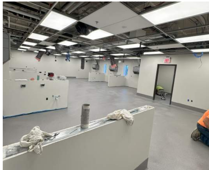
Progress 100's Wing
