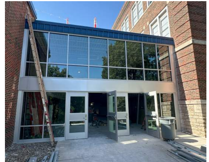
1964 (Area A) Progress
