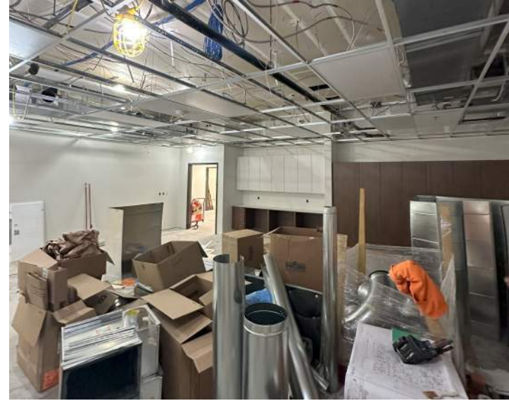
Progress 100's Wing
