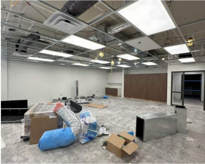
Progress 100's Wing
