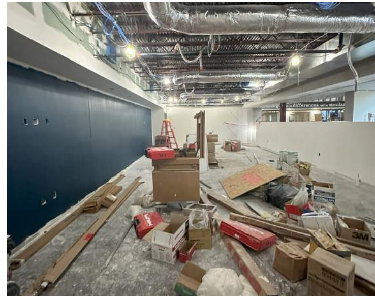
1964 (Area A) Progress
