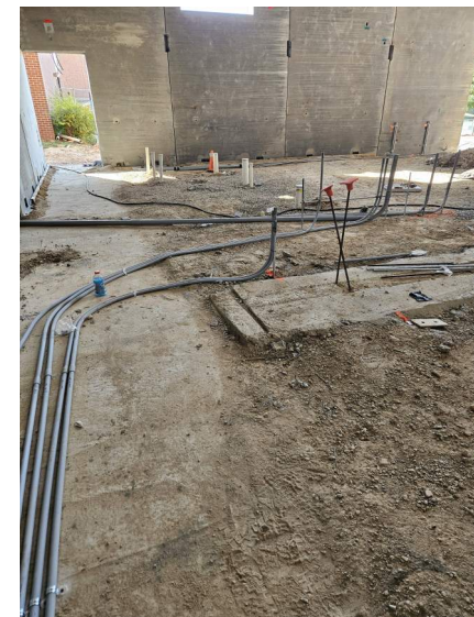
DMS - MEP Under-slab
