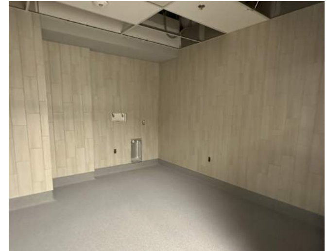
Progress 100's Wing
