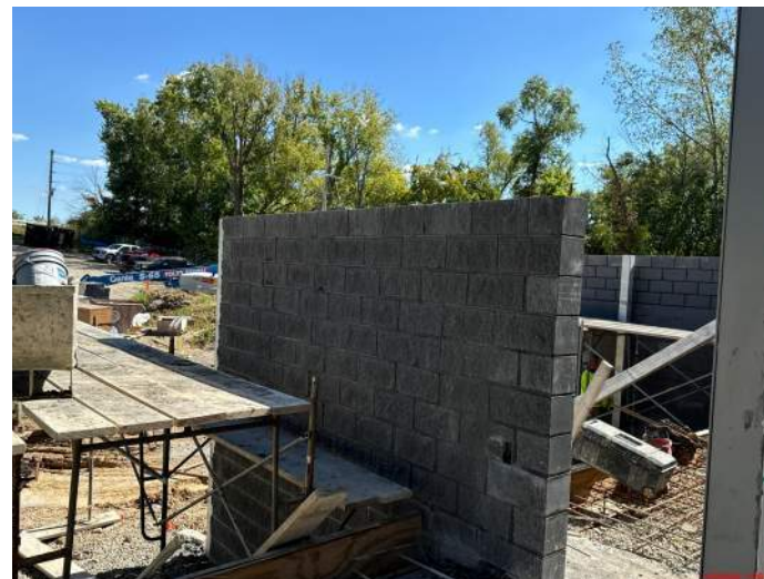
CMU Trash Enclosure
