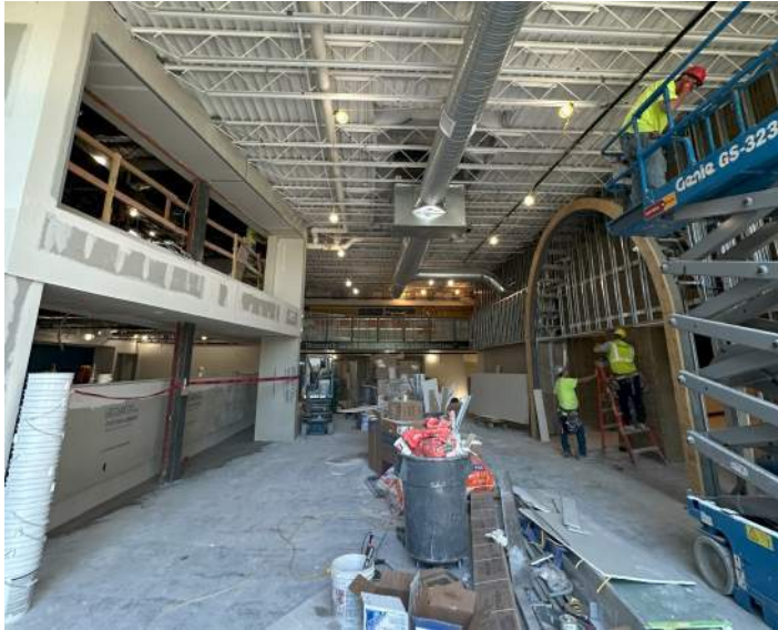
1964 (Area A) Progress
