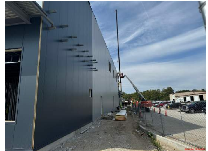
Metal Panels North Wall
