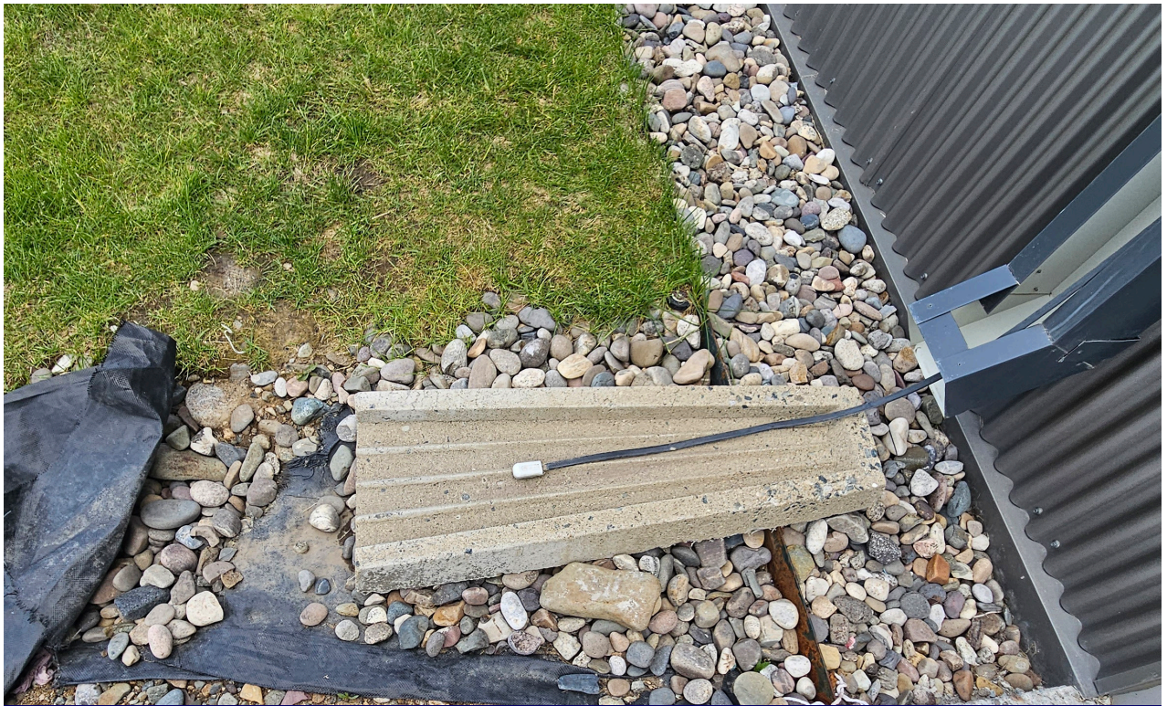
Roof drainage damaging landscaping.
