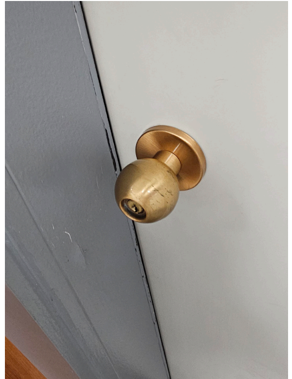
Non-conforming knob-style door hardware.
