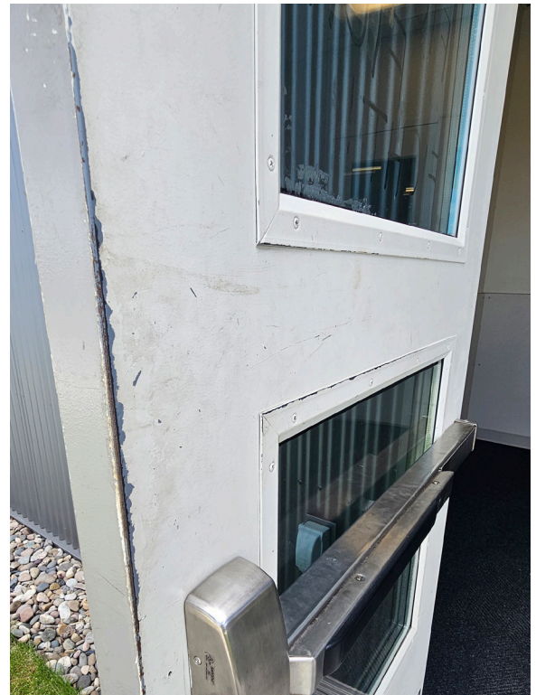
Wear and tear at hollow metal exit door.
