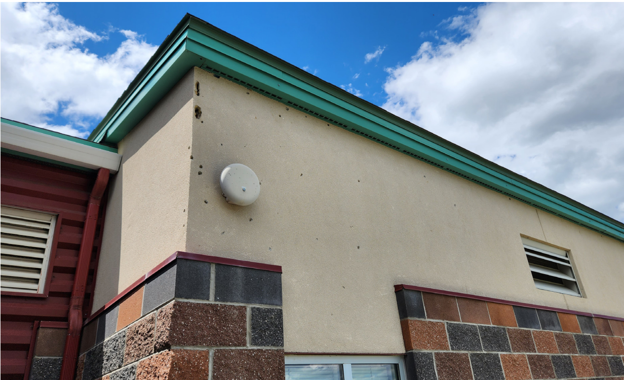
View of damage to the exterior insulation and finish system (EIFS).
