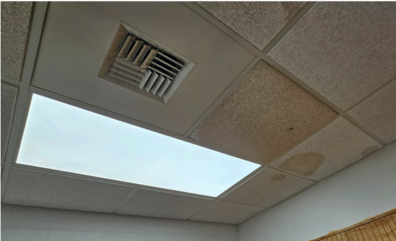
View of damaged ceiling tile.
