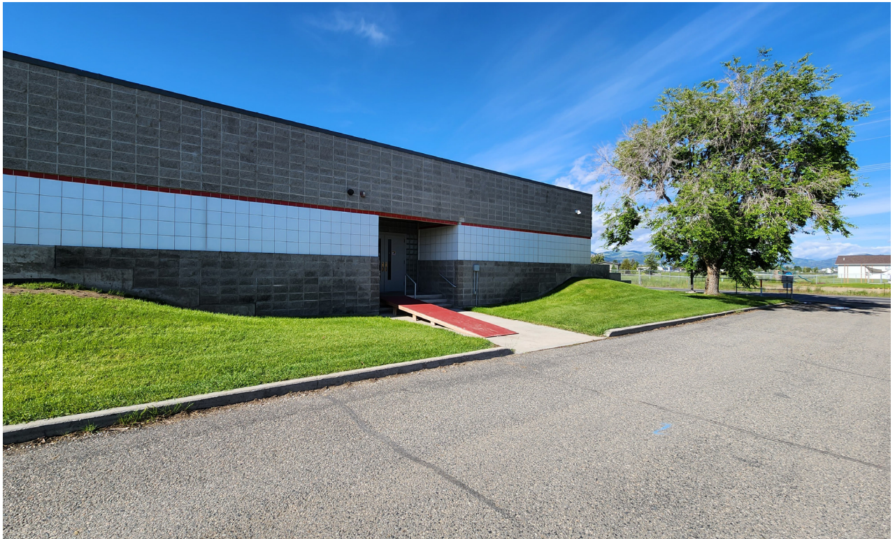
View of northwest exit door with wood-framed ramp.
