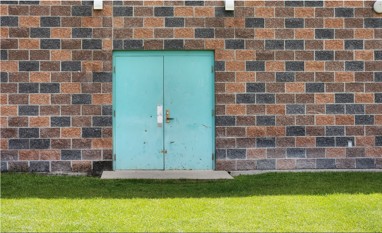
Example view of the condition of the hollow metal doors and frames.
