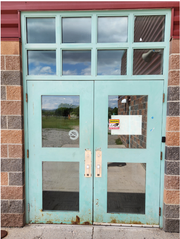
Example views of hollow metal door conditions.
