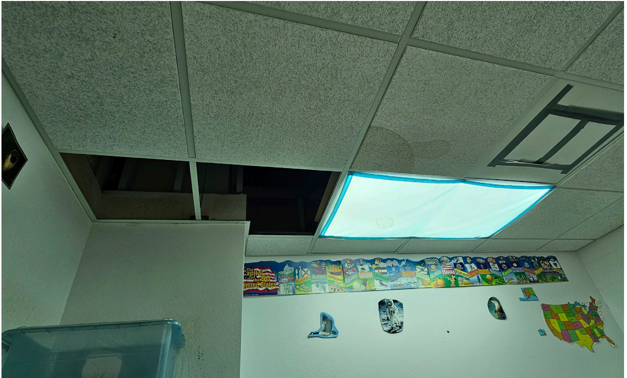
View of damaged ceiling tile.
