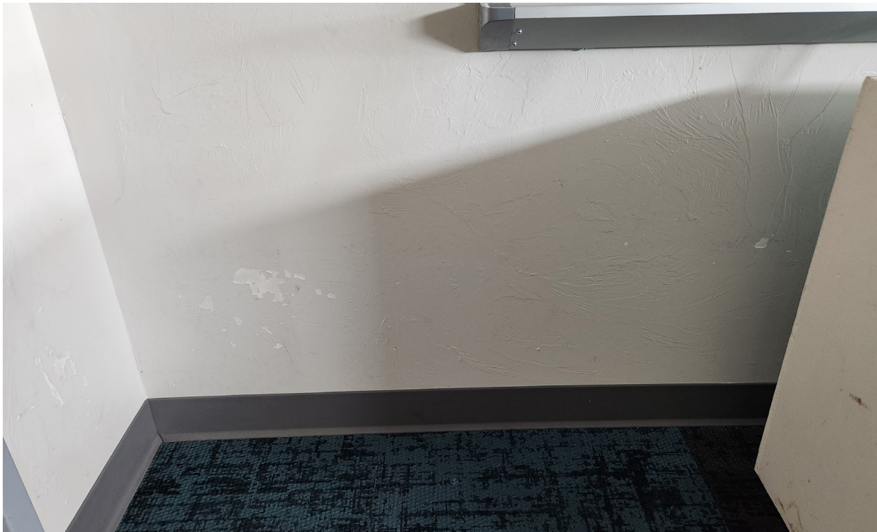
Typical minor damage to drywall finish due to moving furniture.
