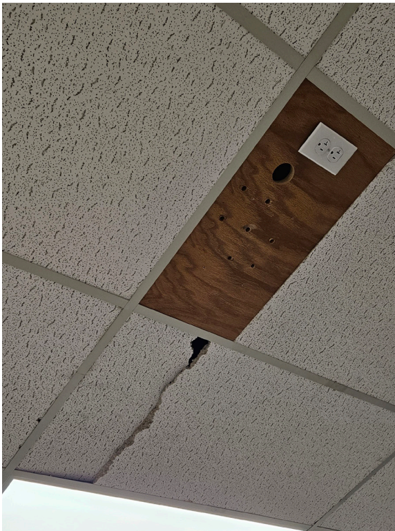
View of damaged ceiling tile.
