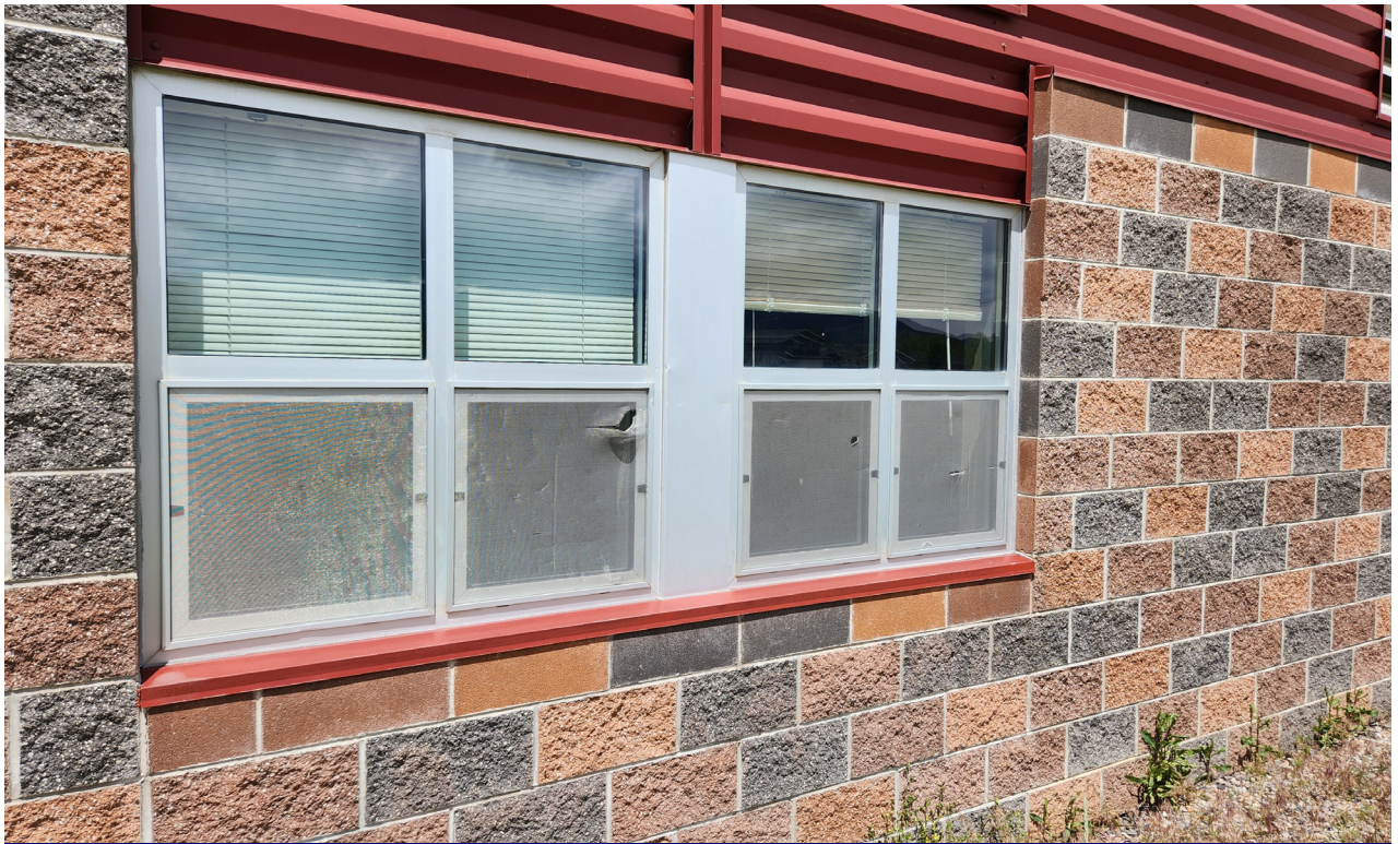
View of damaged exterior window screens.
