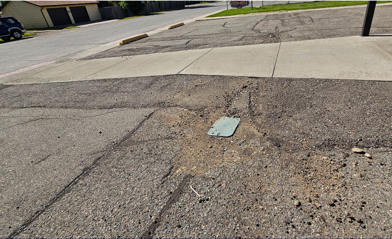
East paved areas, cracked and uneven areas of asphalt.
