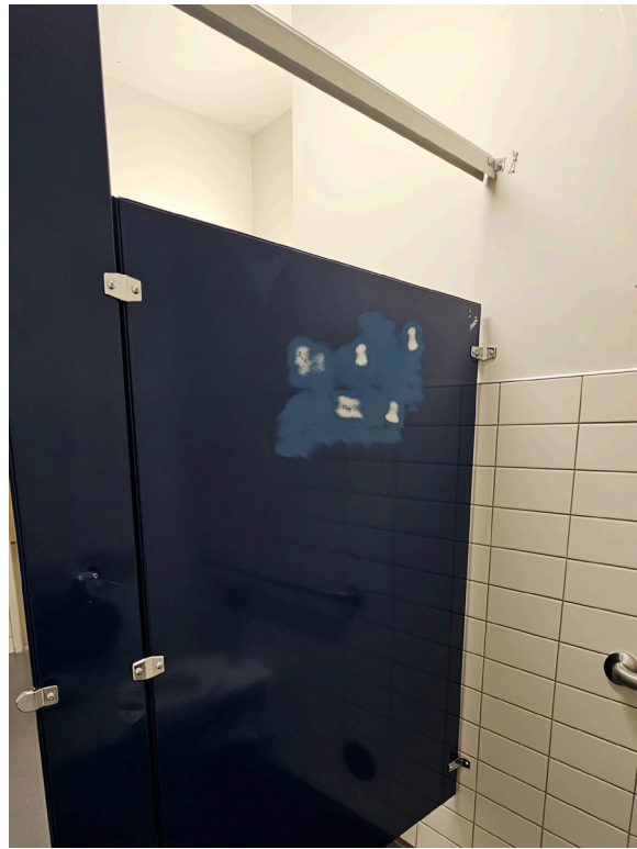
View of damage to toilet partitions.
