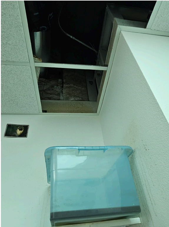
View of damaged ceiling tile.
