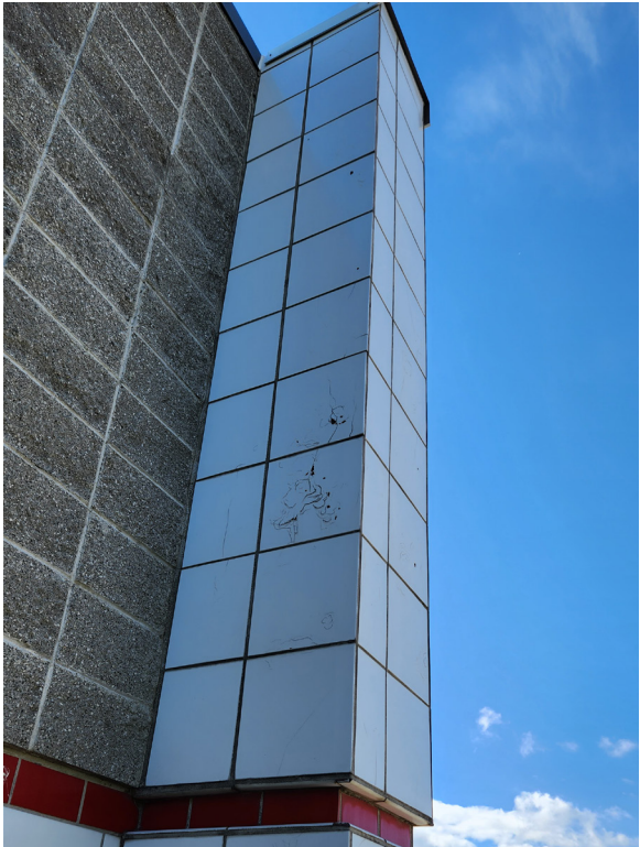
View of damaged glazed tile at main entry.
