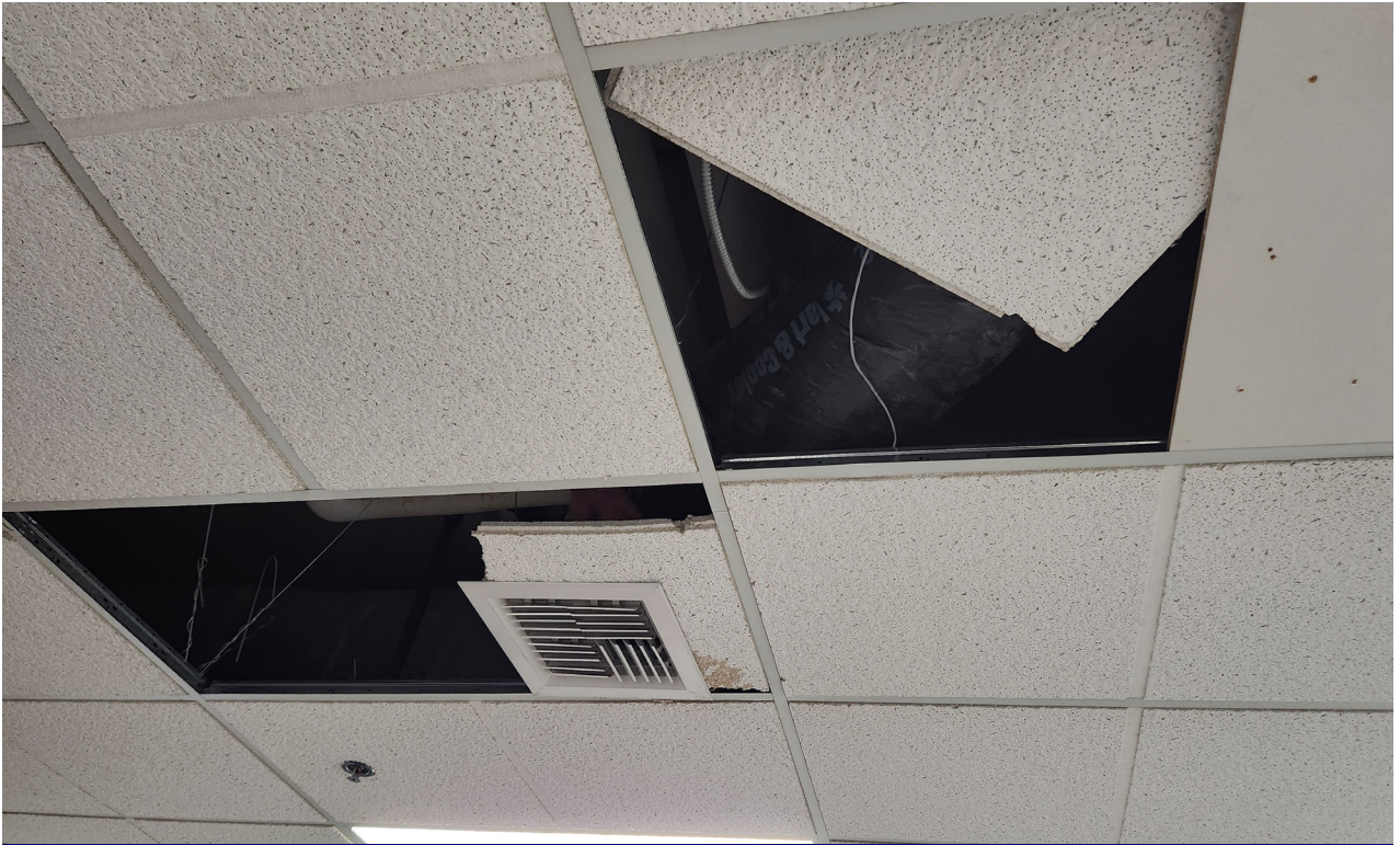
Example of damaged and missing ceiling tiles.
