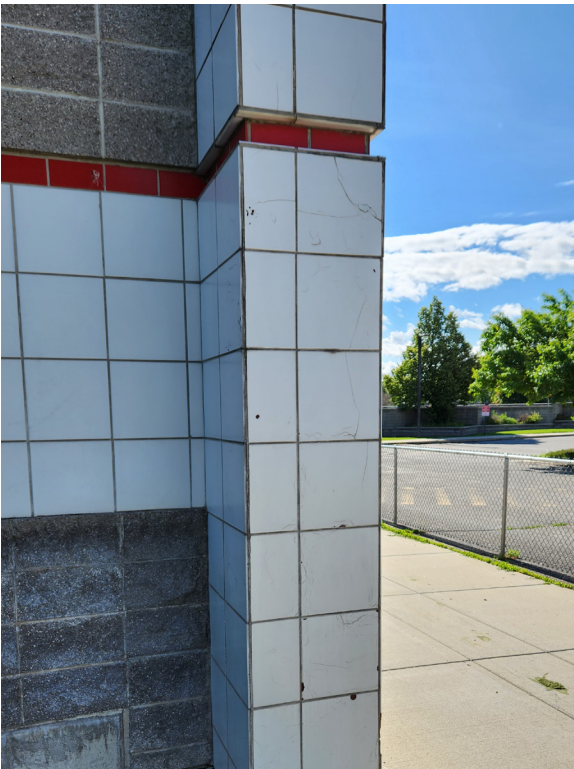
View of cracked and damaged glazed tile at main entry.
