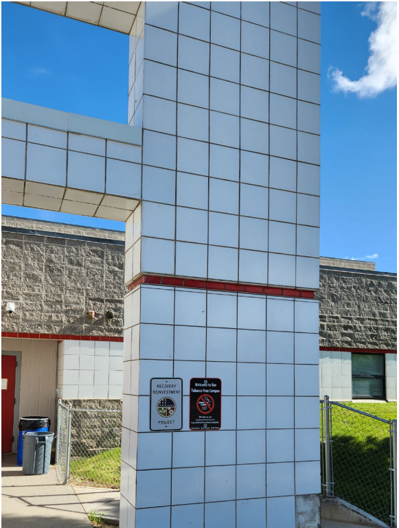
View of damaged glazed tile at main entry.
