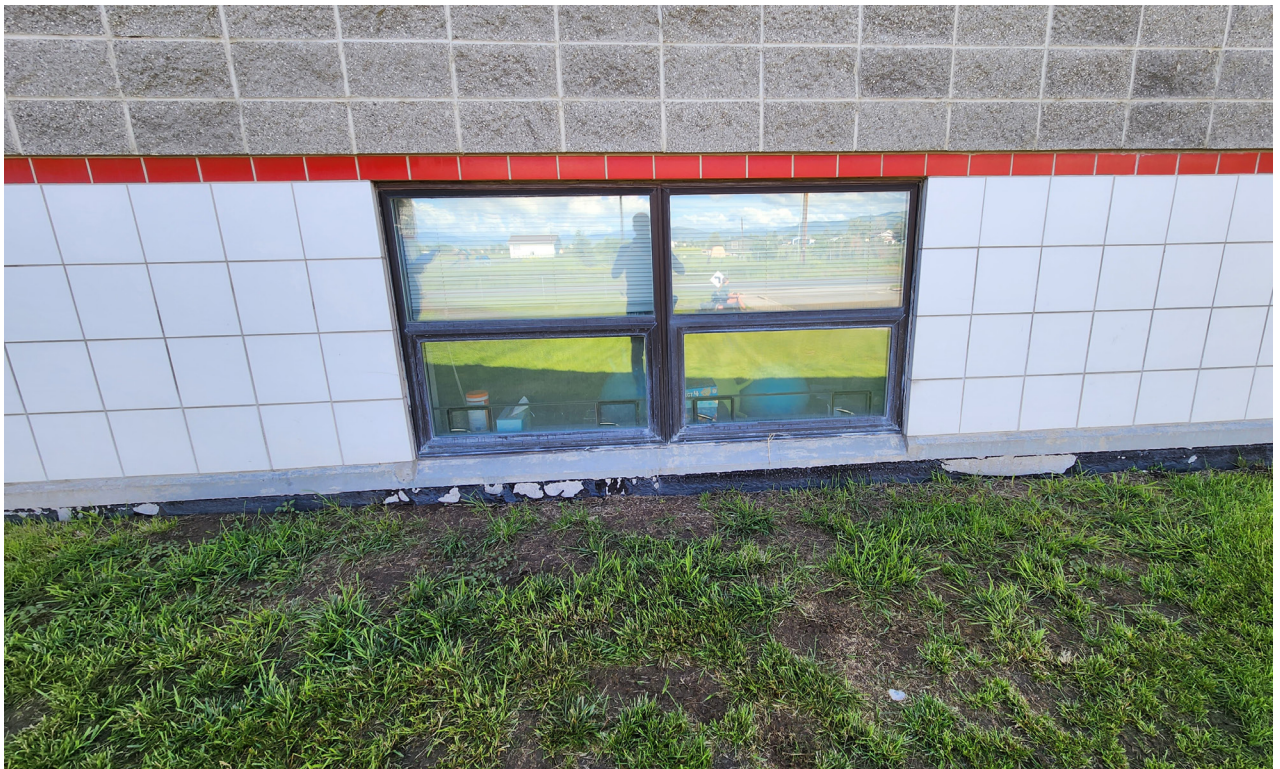
View of foundation and window showing water-proofing peeling from foundation.
