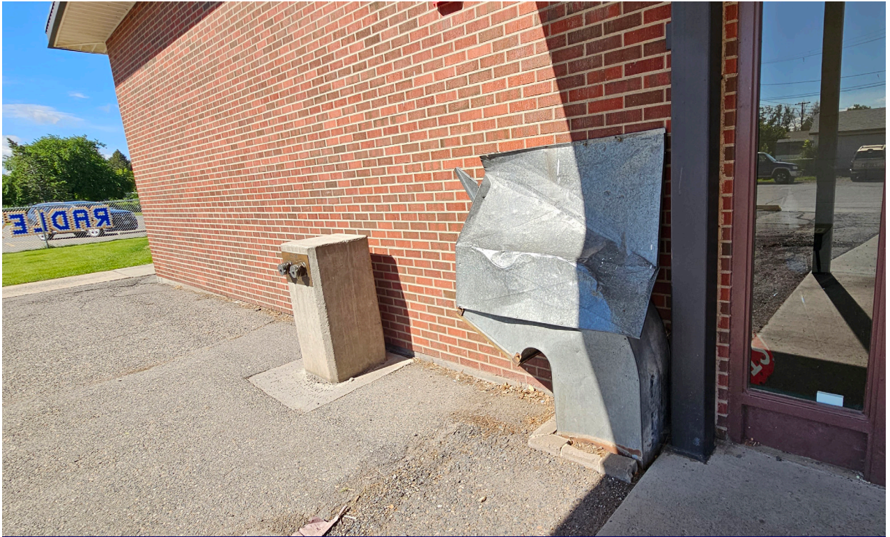
East side of exterior, damaged metal ductwork.
