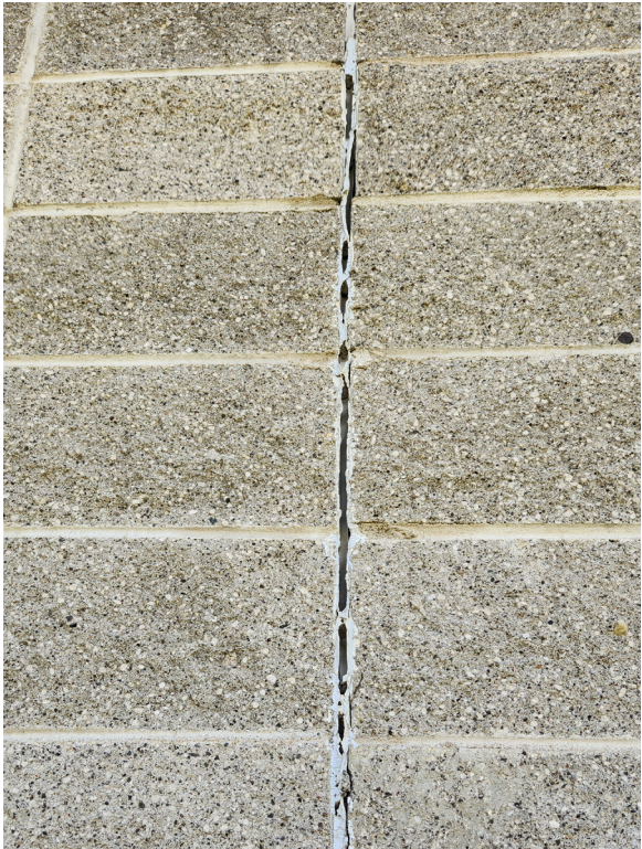
Typical masonry control joint that needs to be re-sealed.
