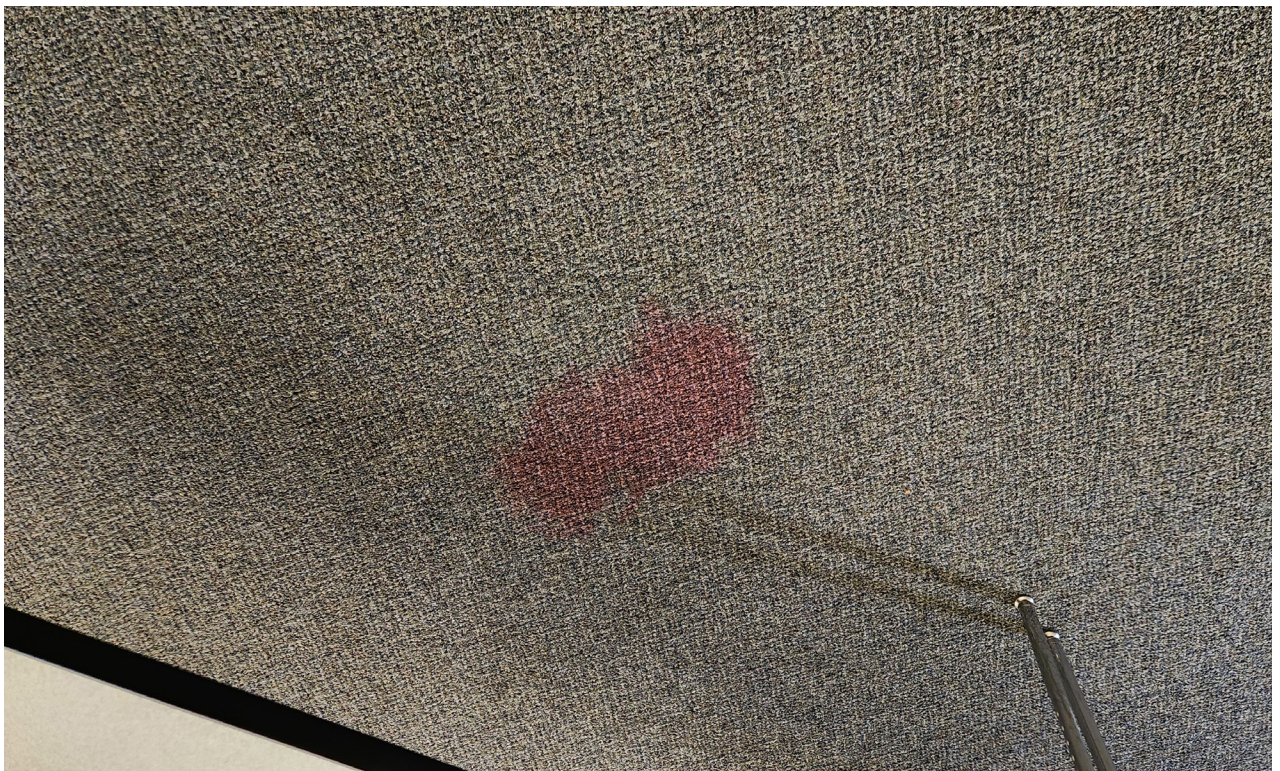
Example view of carpet staining.
