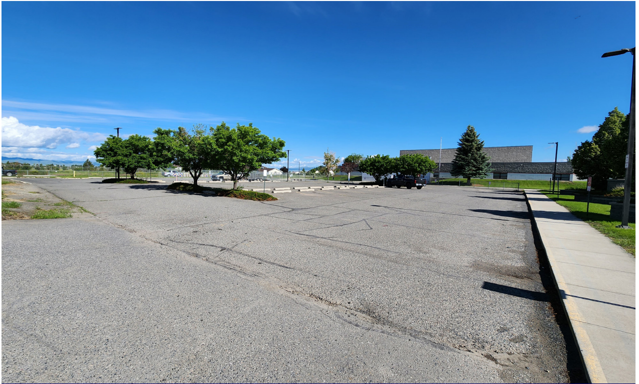
View of south parking lot looking northwest. Note cracking and damage to asphalt.
