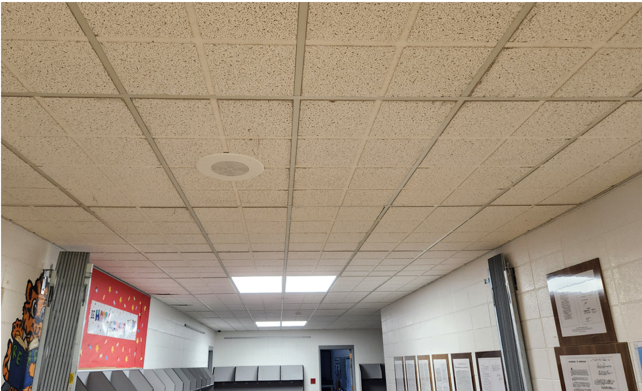
Typical hallway suspended acoustical tile ceiling.
