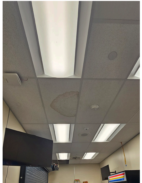
Ceiling tile in Concessions area showing signs of water damage.
