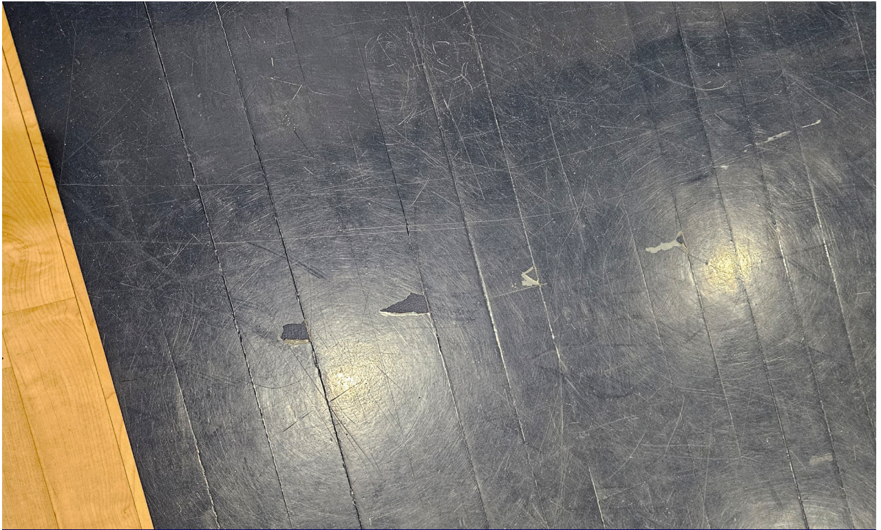
Gym floor finish showing wear and tear.
