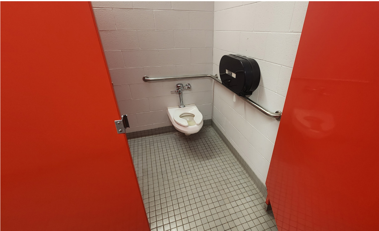
View of typical non-compliant ADA toilet stall.
