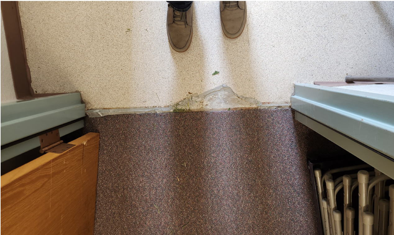
Example of damage at flooring transition.
