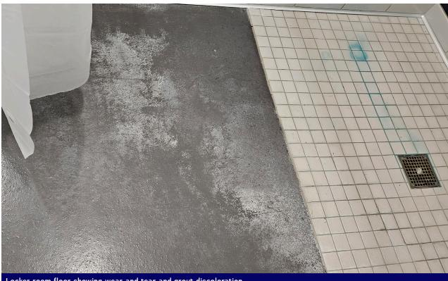
Locker room floor showing wear and tear and grout discoloration.
