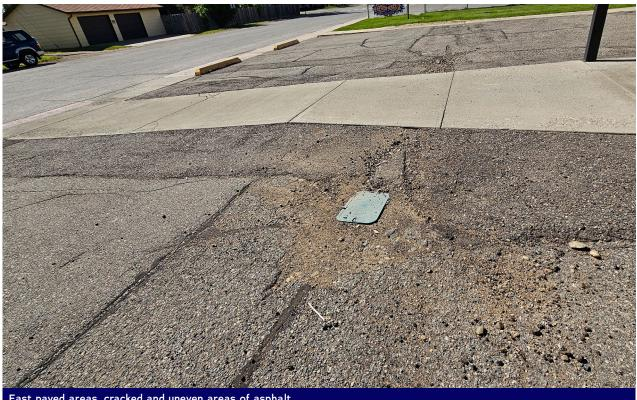
East paved areas, cracked and uneven areas of asphalt.
