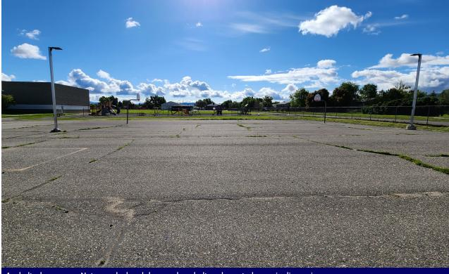
Asphalt play areas. Note cracked and damaged asphalt and sports hoops in disrepair.
