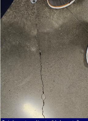
Typical concrete cracking at polished concrete floors.
