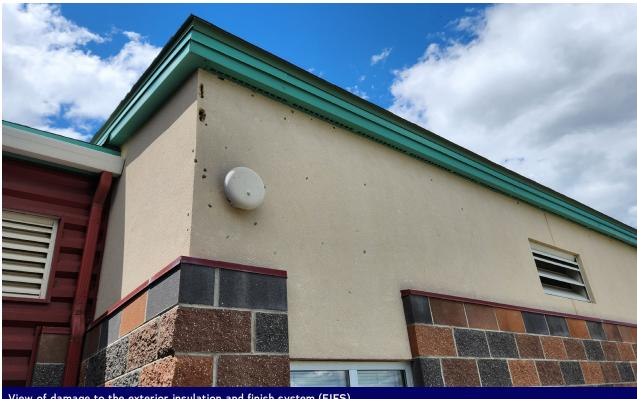
View of damage to the exterior insulation and finish system (EIFS).
