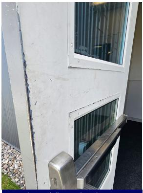
Wear and tear at hollow metal exit door.
