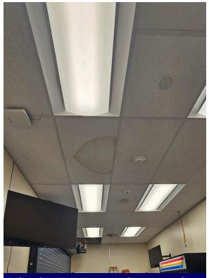
Ceiling tile in Concessions area showing signs of water damage.
