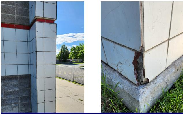
View of cracked and damaged glazed tile at main entry.
