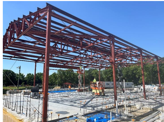
Johnson – steel structure near completion
