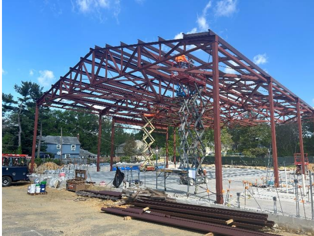
Knight – bolting steel connections
