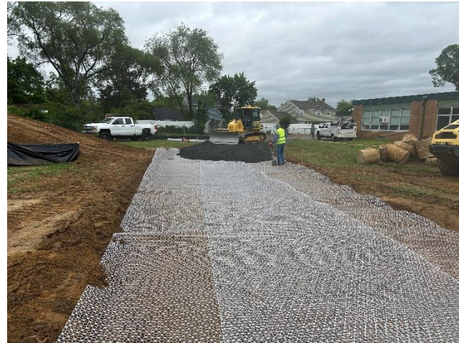
Barton – Geogrid Fabric under access road
