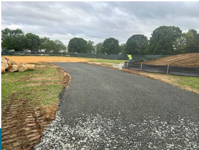
Barton – Stone installed on access road
