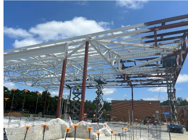
Knight – painting steel structure
