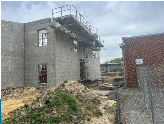
Kingston – CMU walls in progress
