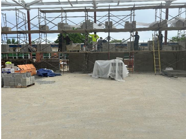
Kingston – CMU walls in progress
