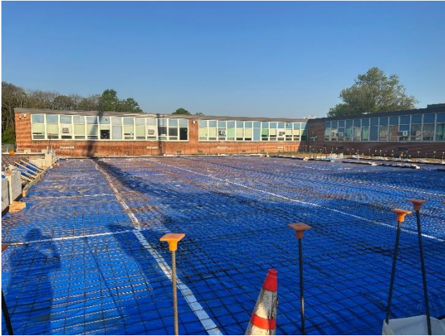
Mann – prep for slab-on-grade
