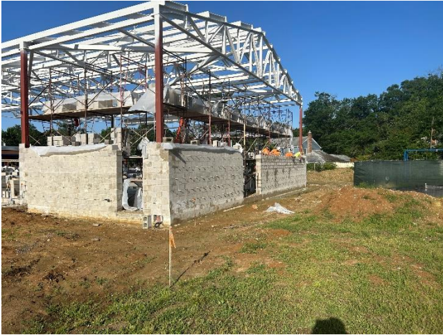
Knight – steel painting and CMU masonry in progress
