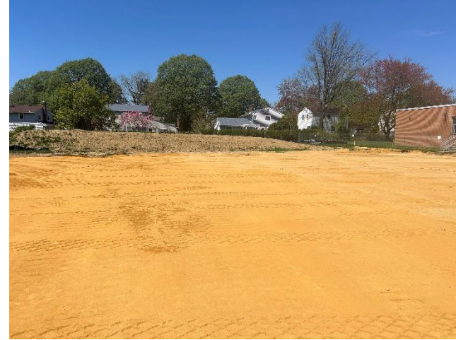
Sharp – constructing building pad
