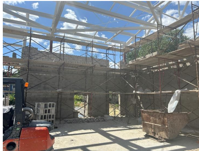
Knight – CMU masonry progress
