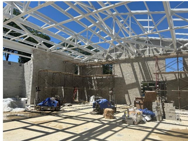
Kingston – CMU walls in progress
