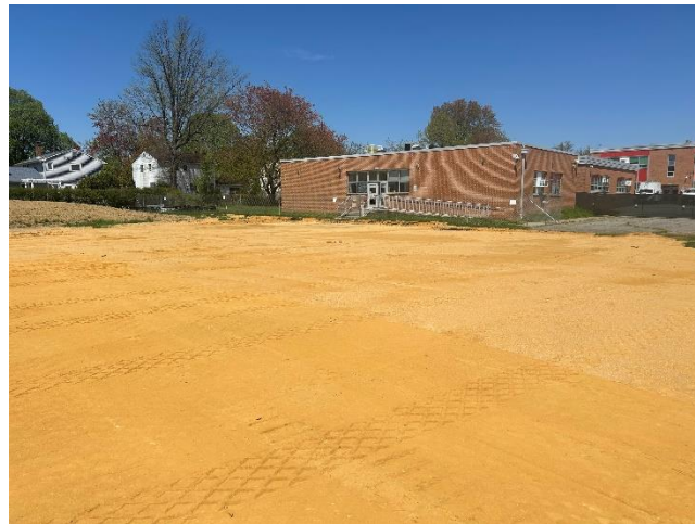
Sharp – building pad complete
