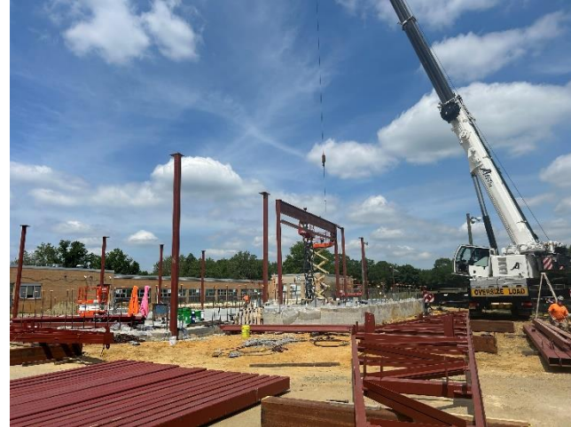
Johnson – structural steel erection
