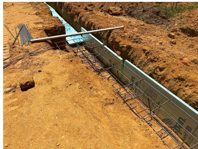
Barton – excavation and rebar for grade beam
