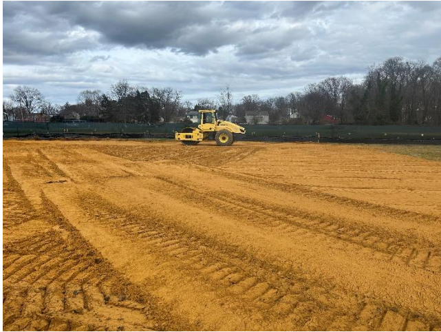
Sharp – constructing building pad
