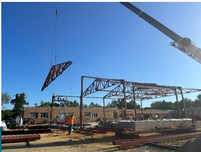
Johnson – setting roof trusses
