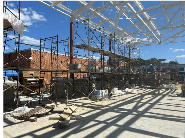
Knight – CMU masonry progress
