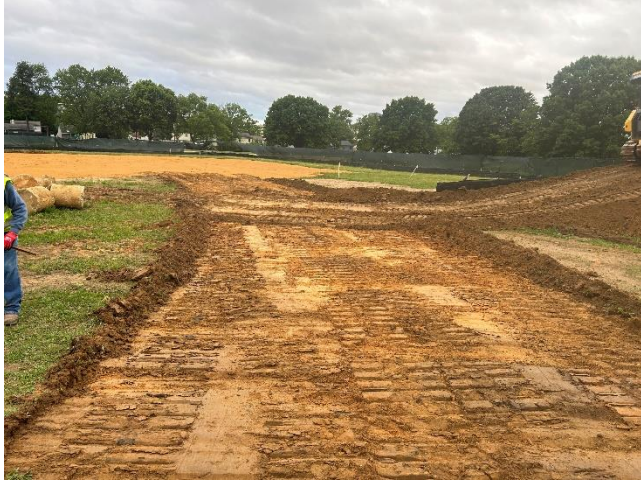
Barton – Stripping Access Road
