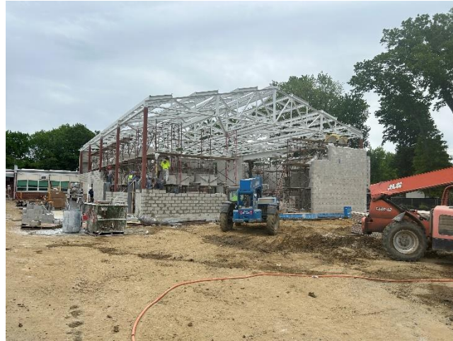
Kingston – CMU walls in progress
