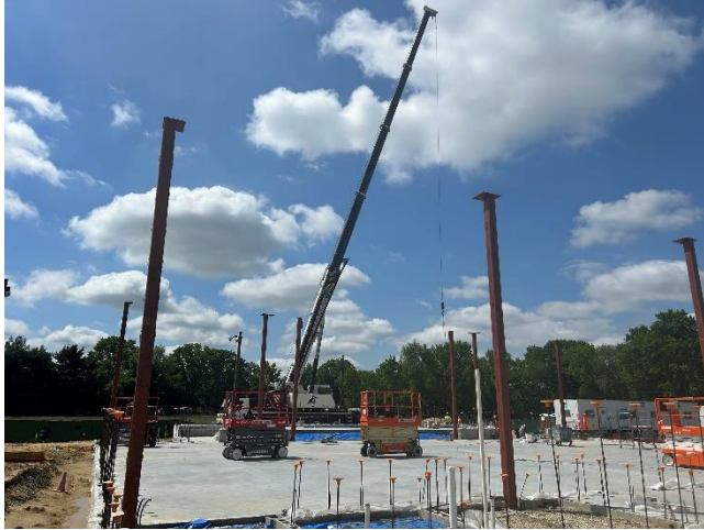
Johnson – setting steel columns
