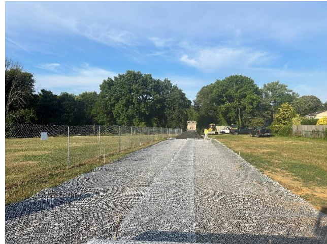
Sharp – geotextile fabric under access road
