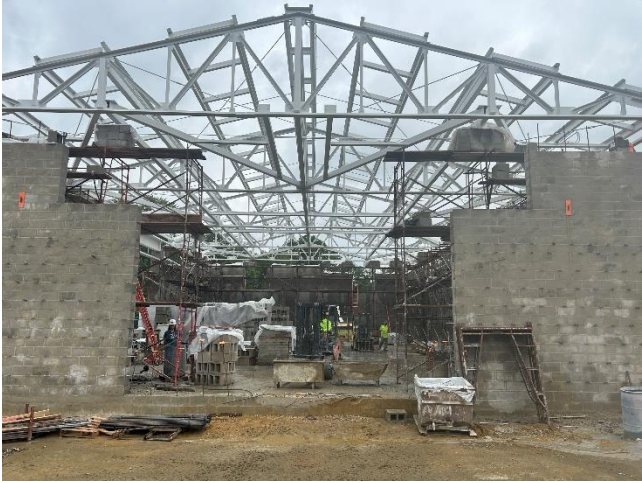
Knight – CMU walls in progress
