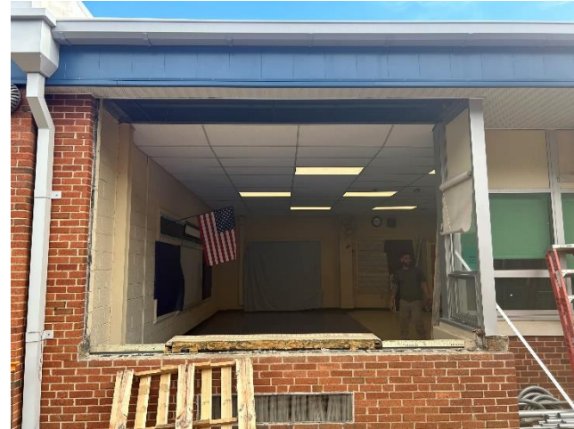
Kingston – demo for connection to existing building
