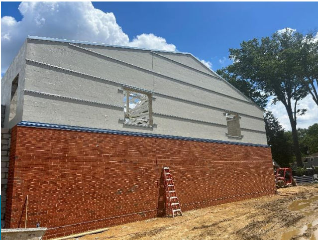
Kingston – brick veneer, beginning wall panels
