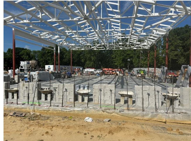
Johnson – beginning block walls
