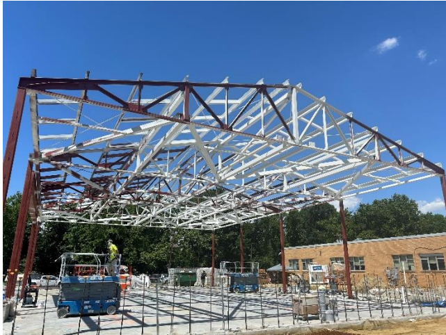
Johnson – painting structural steel
