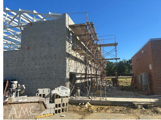
Knight – CMU walls in progress
