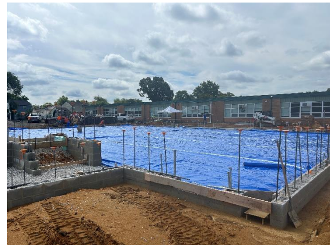
Barton – prepped for floor slab
