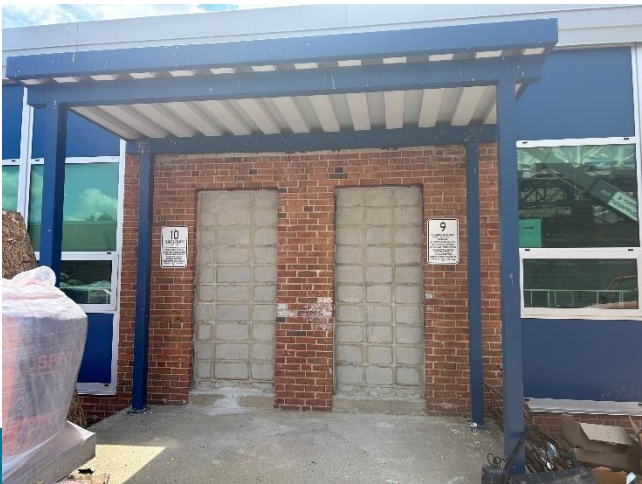
Knight – infill of existing door openings
