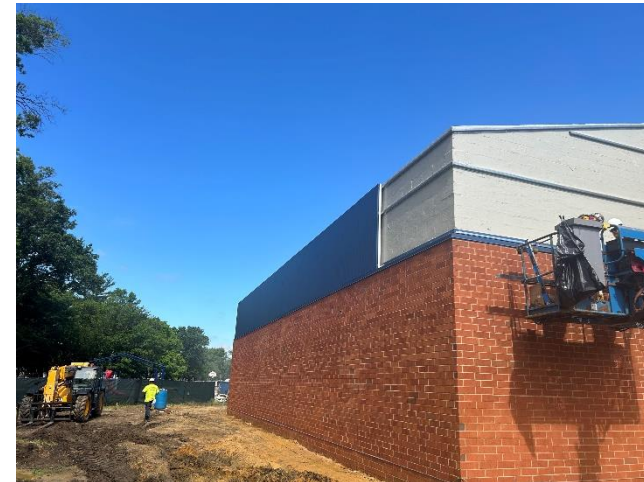
Kingston – brick veneer completed, wall panels underway
