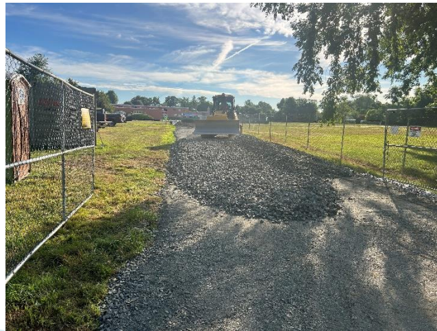
Sharp – spreading stone on access road
