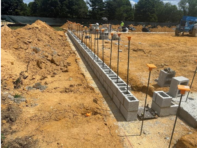
Barton – Foundation walls being constructed
