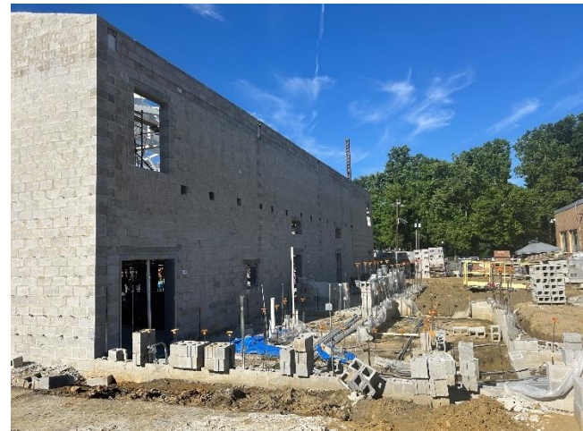
Johnson – block wall construction
