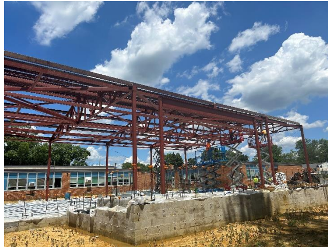
Mann – steel near completion
