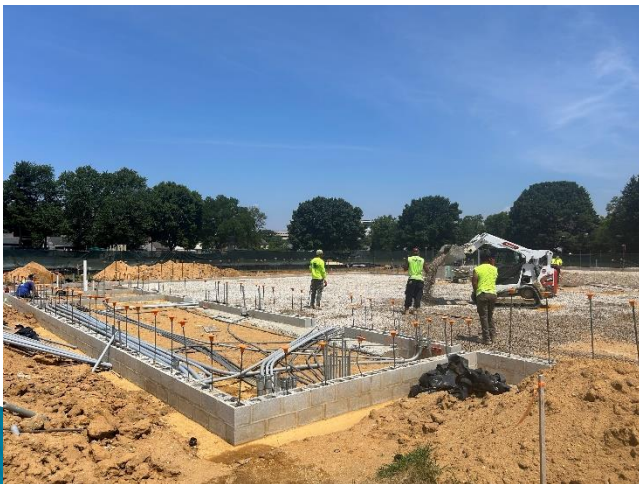
Barton – Stone under slab on grade
