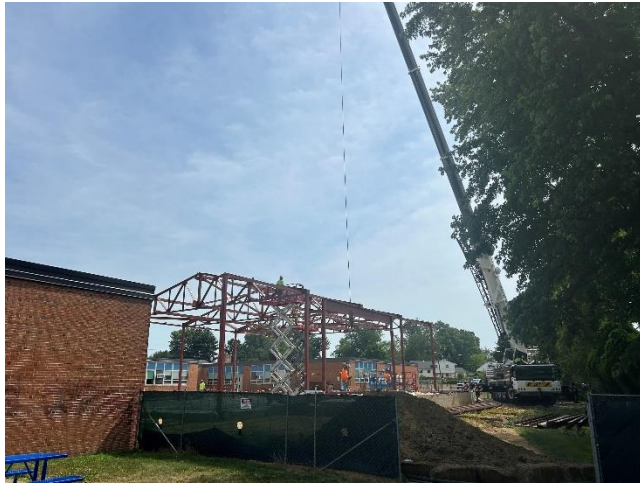
Mann – structural steel erection in progress
