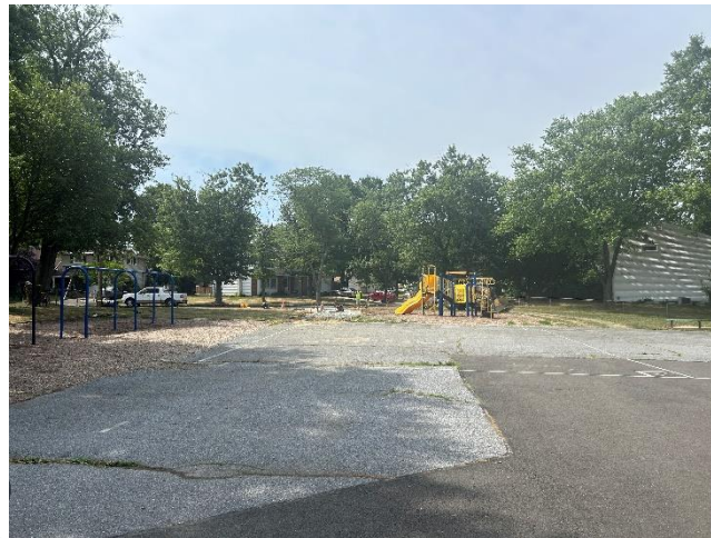
Mann – playground reconstruction underway
