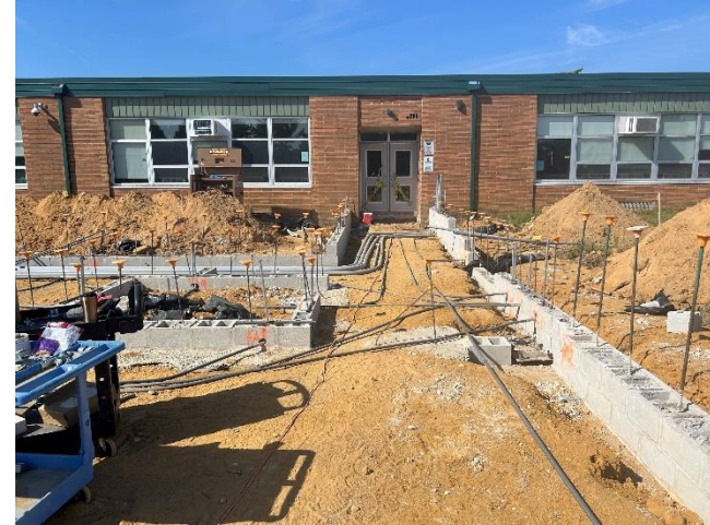
Barton – Underground conduits and foundations
