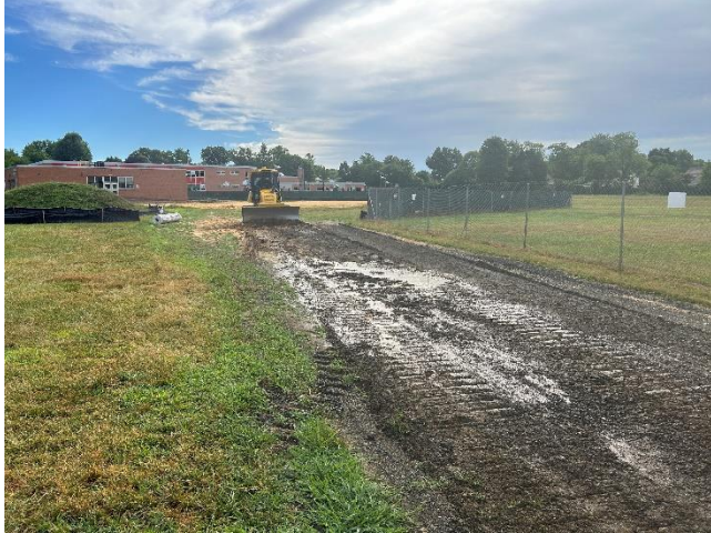
Sharp – grading new access road
