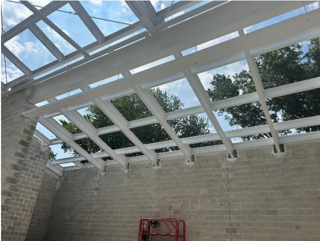
Kingston – steel structure (low roof area)
