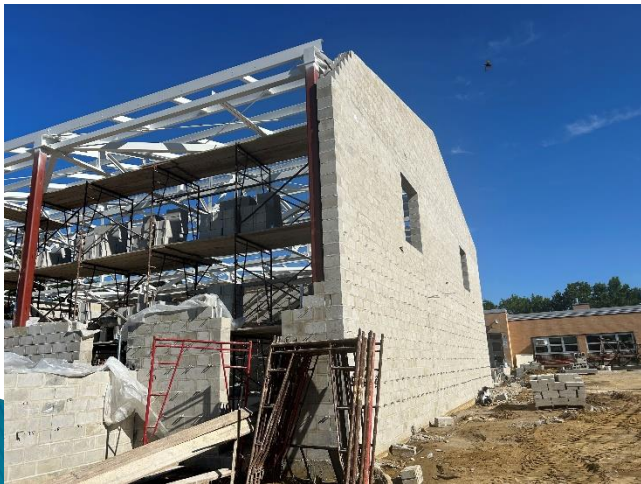
Johnson – block wall construction
