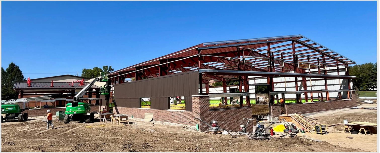
Above: a photo of the overall progress at the Yahara Site of the Maintenance Building as the metal wall panels go into place
