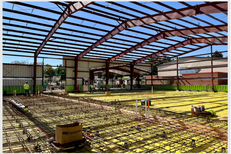
Above: a photo inside the Maintenance Building prior to the first slab-on-grade pour in the shop space
