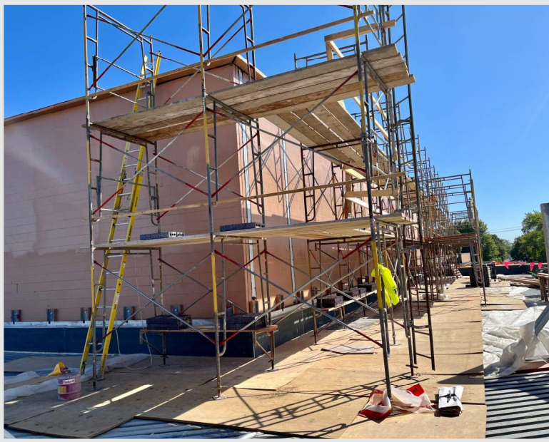
Bottom Left: a view on the low roof of the River Bluff addition as scaffolding is set in preparation for brick masonry to begin
