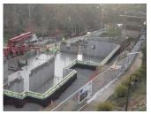
Work continues on the new music building, but with a much slower rate of progress. Over the last three months, 45-plus "weather days" have delayed installation of some foundations, walls, and the lower-level concrete floor. Installation of the structural steel for the upper floor is scheduled to begin in the next 2-3 weeks.
