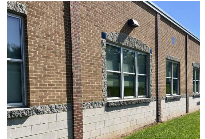
● Ext. Walls - Missing/Cracking sealant at expansion joints
