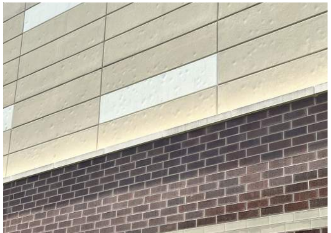
Ext. Walls - Some cracking and spalling
