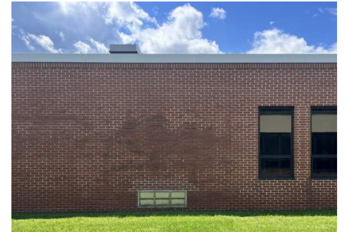
● Ext. Walls - Masonry shows signs of aging; Staining; Flood control
