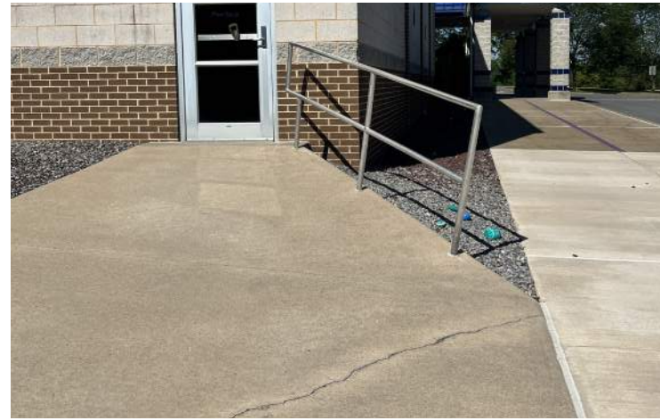
● Ext. ADA - Slight cracking
