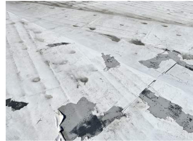
● Roof - TPO Peeling; EPDM
