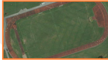
Poor Drainage at Varsity Soccer Field
