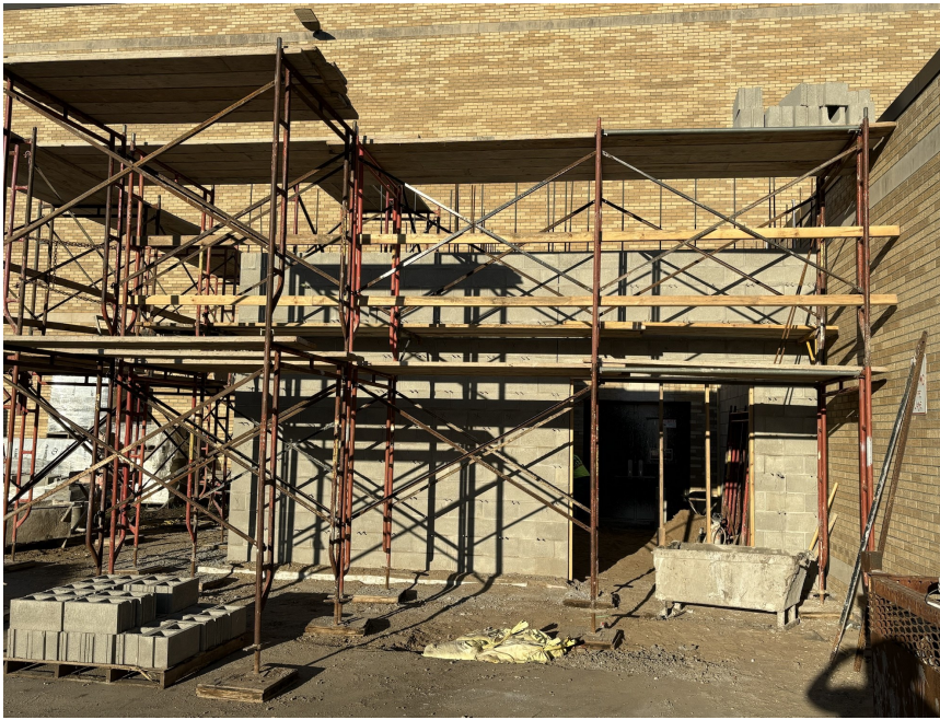
ELEVATOR ADDITION MASONRY
