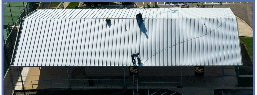
TENNIS BUILDING RENOVATION
