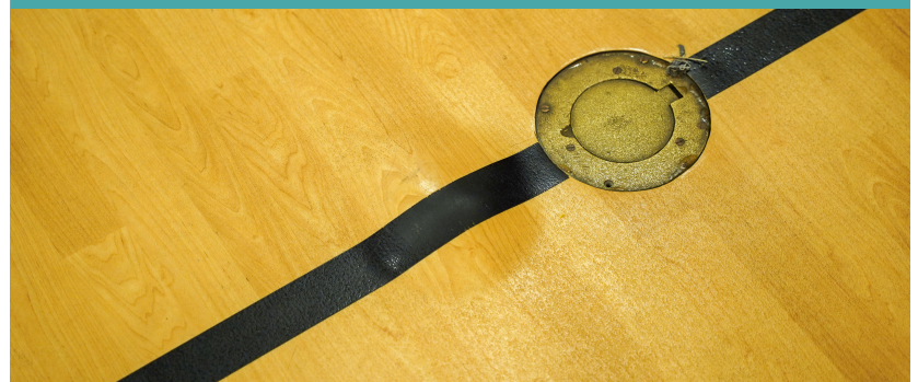
FLOORING IS WARPED
