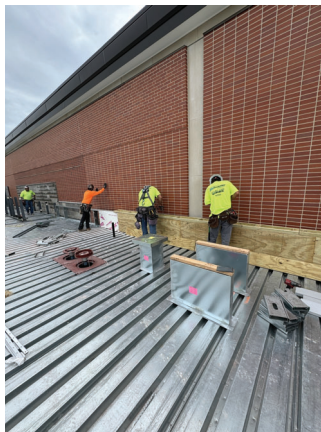
Roof Blocking and Sheathing
