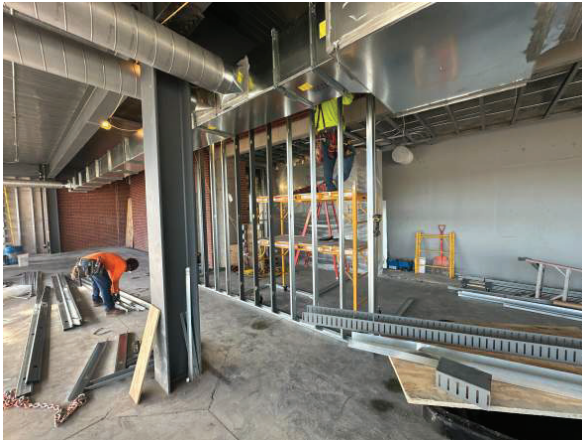
Interior Wall Framing
