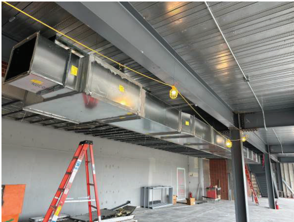
Lower Level Duct Work
