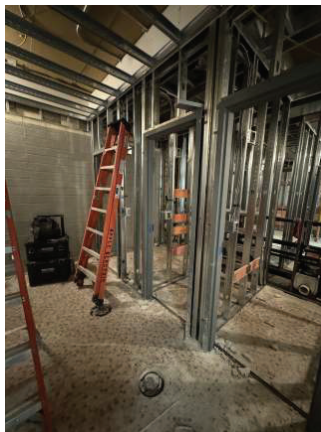
Restroom Wall Framing
