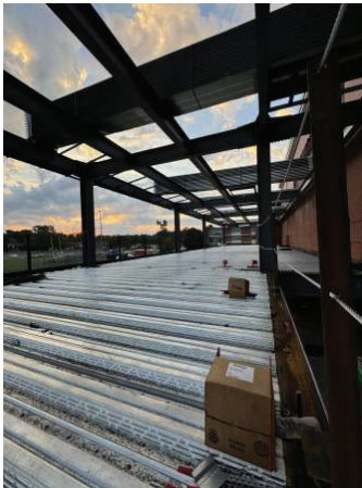
2nd Level Steel Deck
