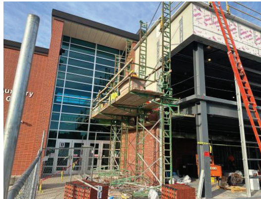
East Wall Brick Install
