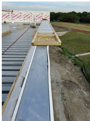
Roof Parapet Blocking
