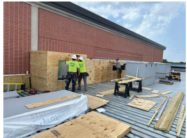
Roof Dog House Wood Blocking
