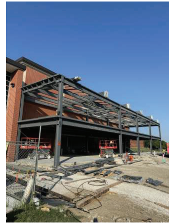
Columns and Beams Set
