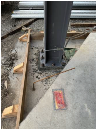
Grout Column Base Plates
