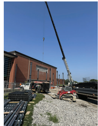
Building Addition Set Columns
