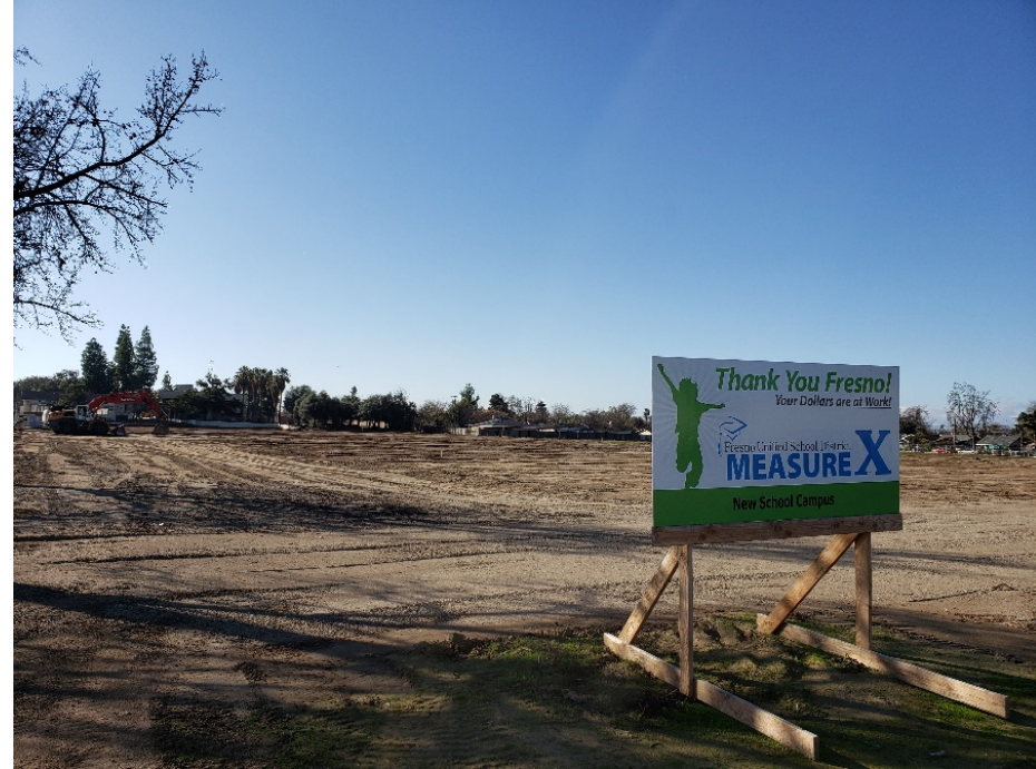
Cleared site, ready for development
