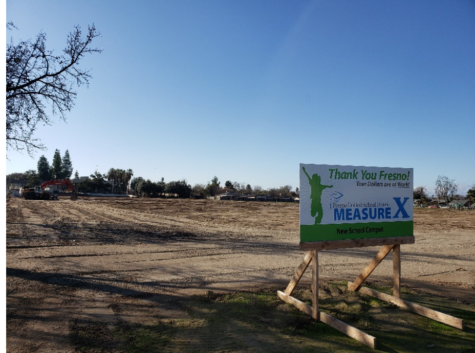
Cleared site, ready for development
