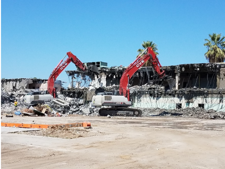
Demolition of former county juvenile detention center
