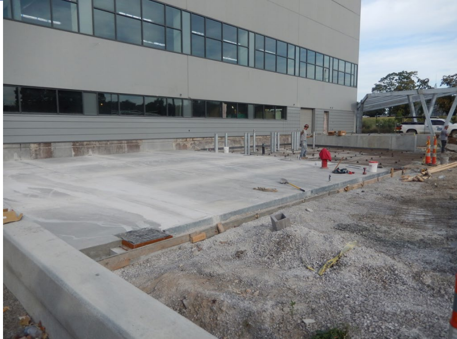
Concrete Slab at Dumpster and Dock Area
