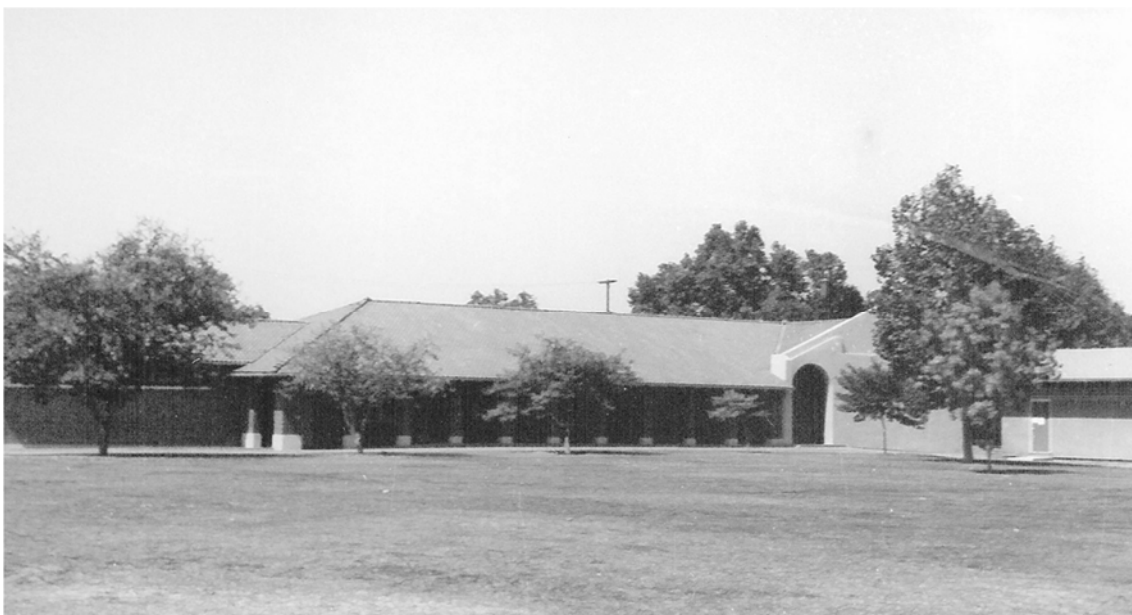
Two classroom wings constructed in 1927
