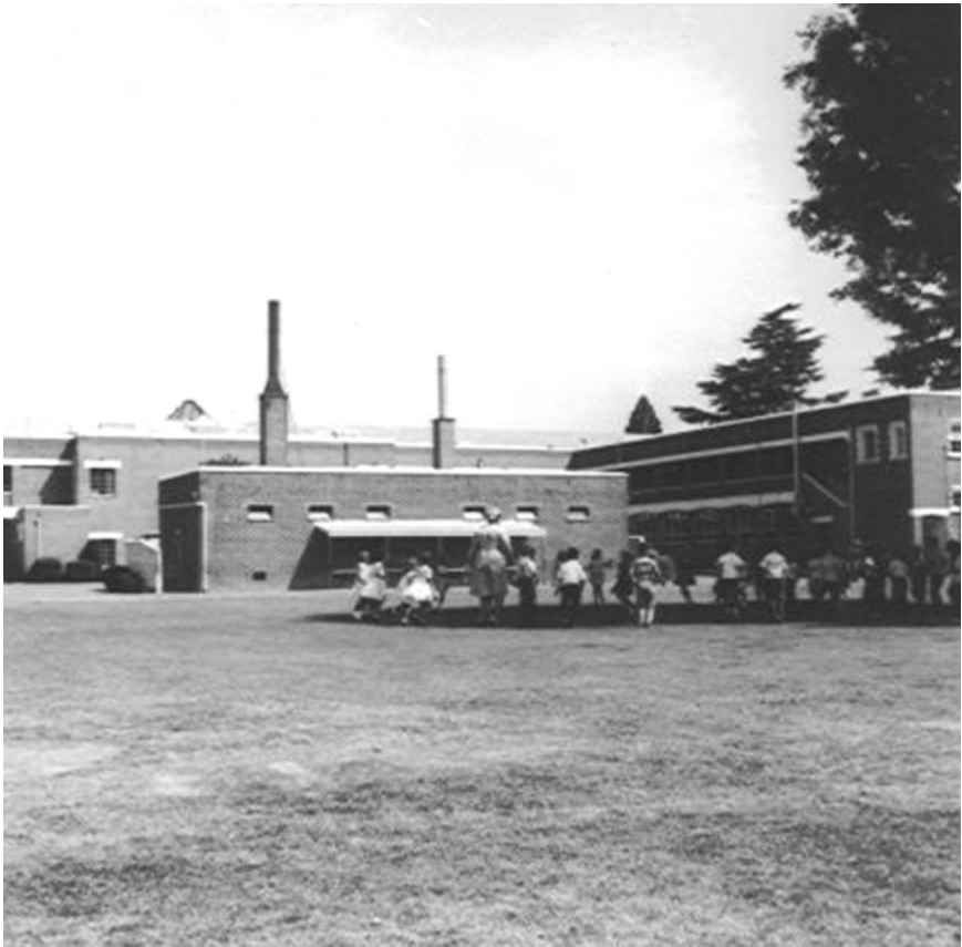
Rear of the school and the toilet buildings prior to demolition
