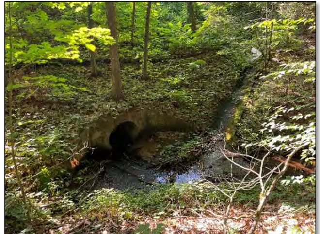
Photo 2: A culvert near the southeastern corner of the Site.
