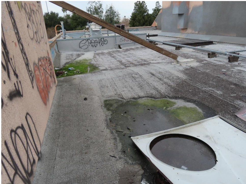
Area to Perform Roof Maintenance
