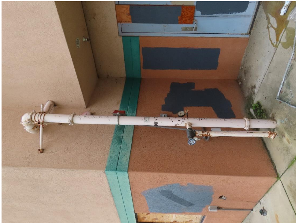
Fire Riser No Shut Off
