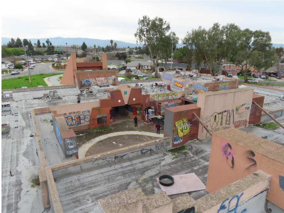
Shot from Gym Roof Ladder
