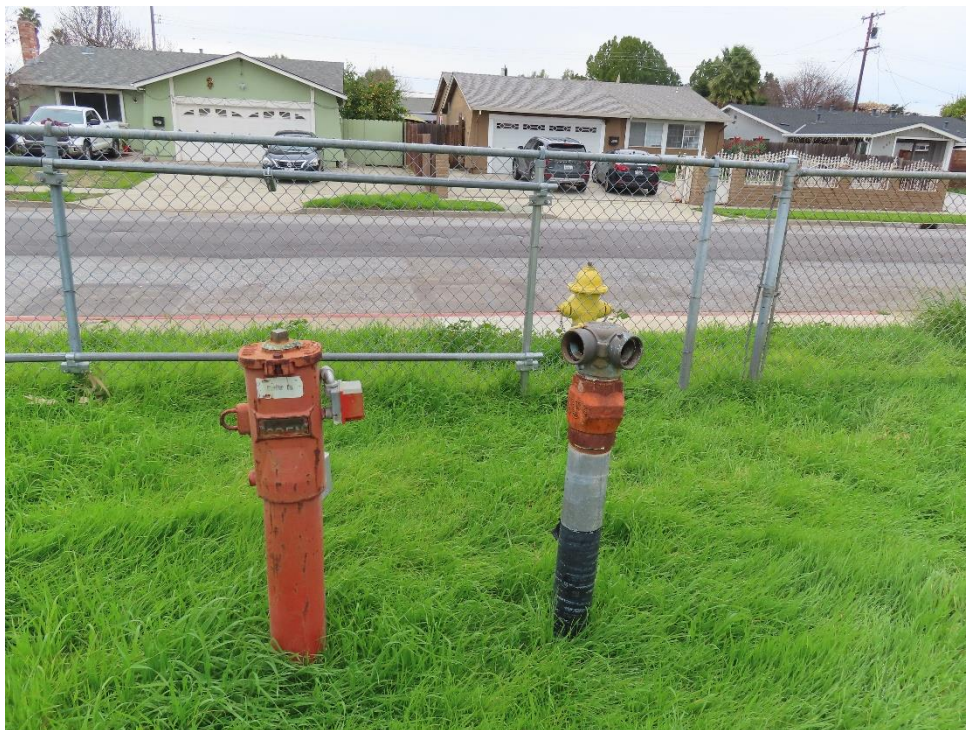
Existing PIV, Hydrant, Fire Dept. Connection
