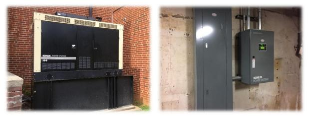
100KW Emergency Generator and Automatic Transfer Switch
