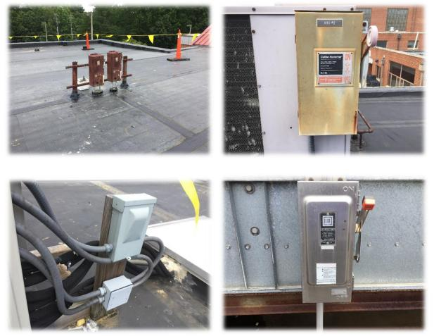
**Disconnect Switches Serving Roof Mounted HVAC Equipment**
