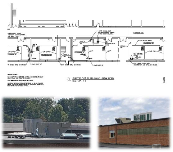
Variable Refrigerant Flow Condensing Units and 100% OA Ventilation Unit (2017)
