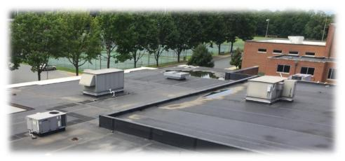
Dual Temperature Air Handling Units and Packaged Rooftop Unit (2009)
