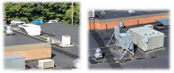
Packaged Rooftop Air Conditioning Unit (2007) Packaged Rooftop VAV Air Conditioning Unit (2007)
