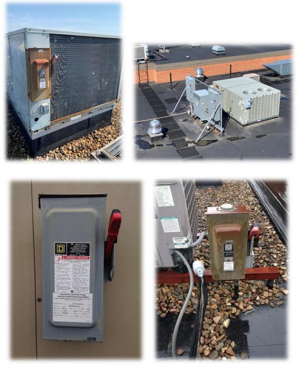
Disconnect Switches Serving Roof Mounted HVAC Equipment
