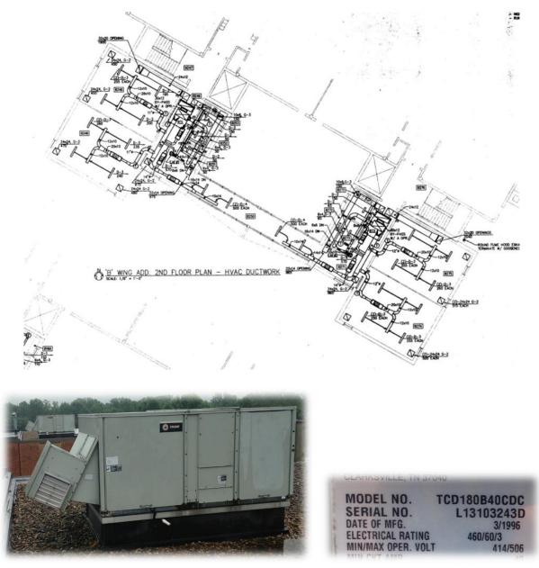
Packaged Rooftop Air Conditioning Unit Serving Hot Water Induction Boxes (Typical of 2) (1996)
