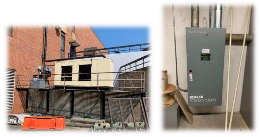
250KW Emergency Generator and Automatic Transfer Switch
