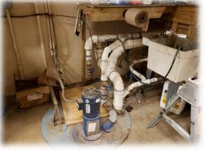
Sewage Lift Station in Main Boiler Room Sewage Lift Station in Mechanical Room Below Stage
