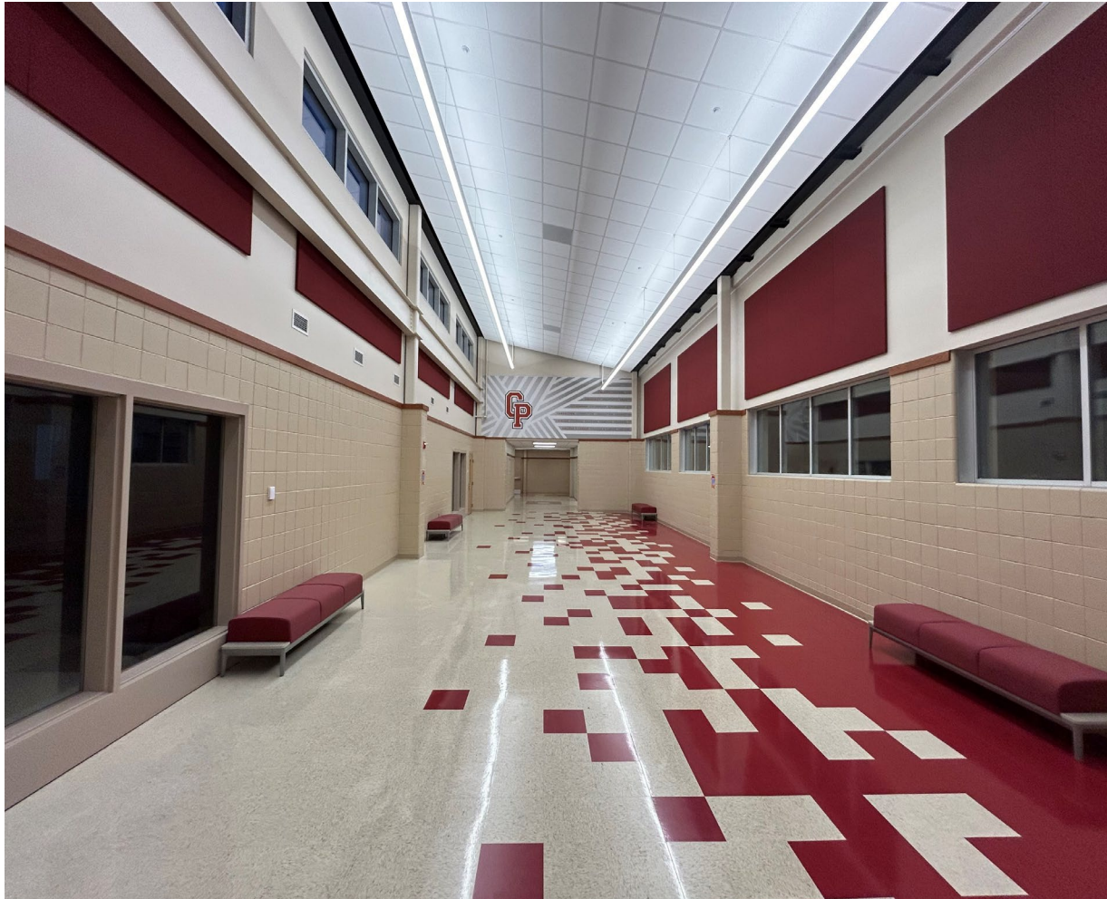
Completed Clerestory Hallway
