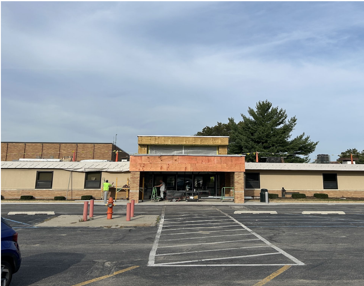
New Clerestory/Roofing Progress
