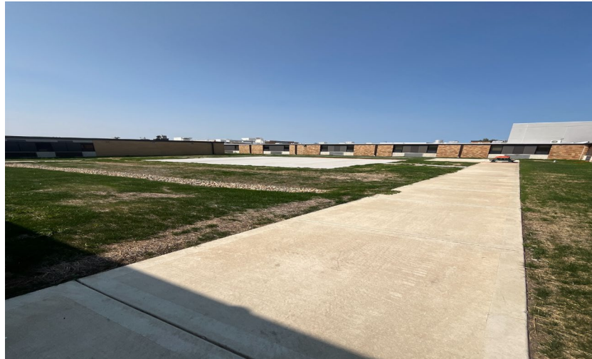
Courtyard Landscaping Progress
