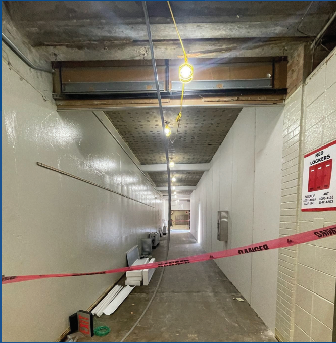
TEMPORARY PARTITION IS IN PLACE
