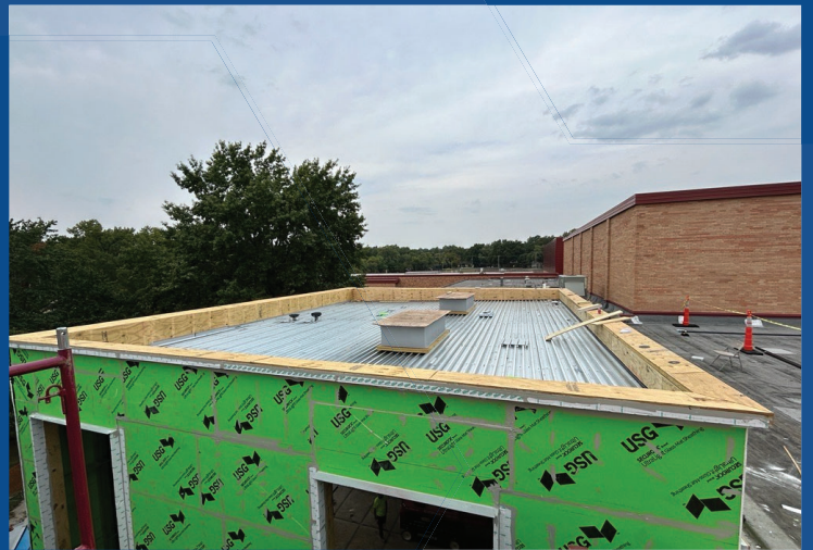
Parapet framing & roof blocking are complete.
