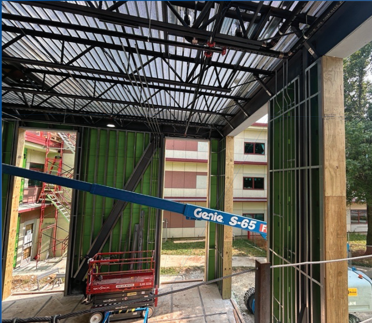
MEP overhead & in-wall rough-in are in progress.
