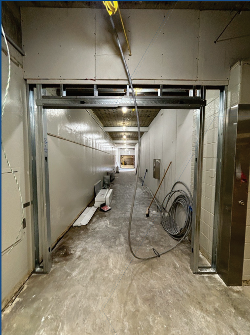
Walls and openings are framed on the Ground Floor
