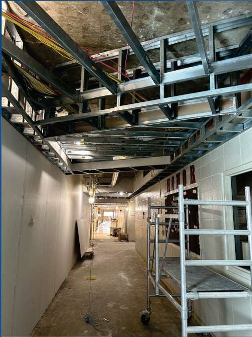
Hardlids and soffits are framed in the 1st Floor Hallway
