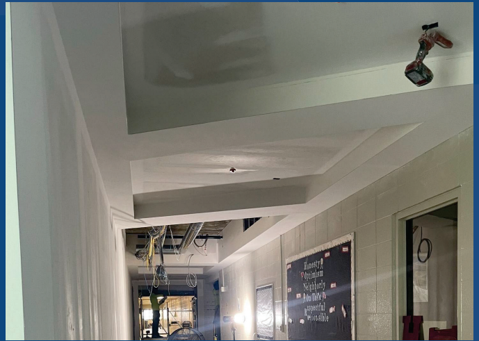
Hardlids are complete in the hallways and grid is being installed, Painting has begun
