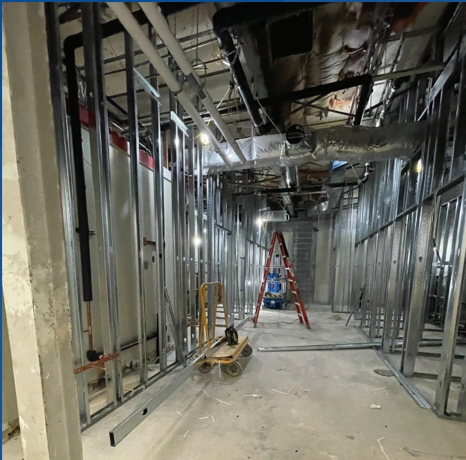
WALLS HAVE BEEN FRAMED IN THE RESTROOM
