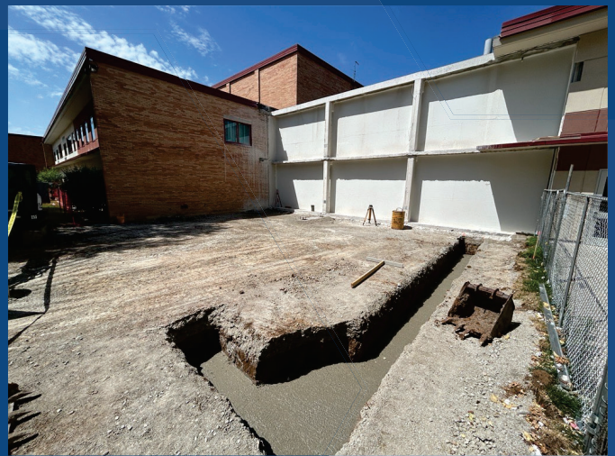
Footings for the addition have started
