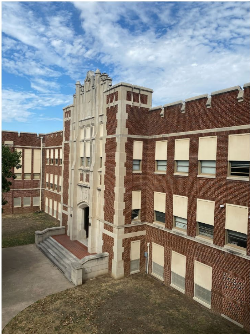
NON-ADA COMPLIANT & UNSECURED MAIN ENTRY AND DAYLIGHTING OBSCURED BY BOARDED WINDOWS
