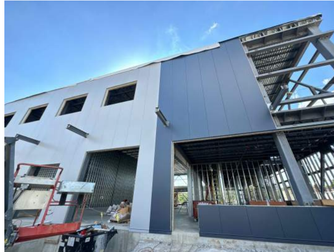
Metal Panels East Wall
