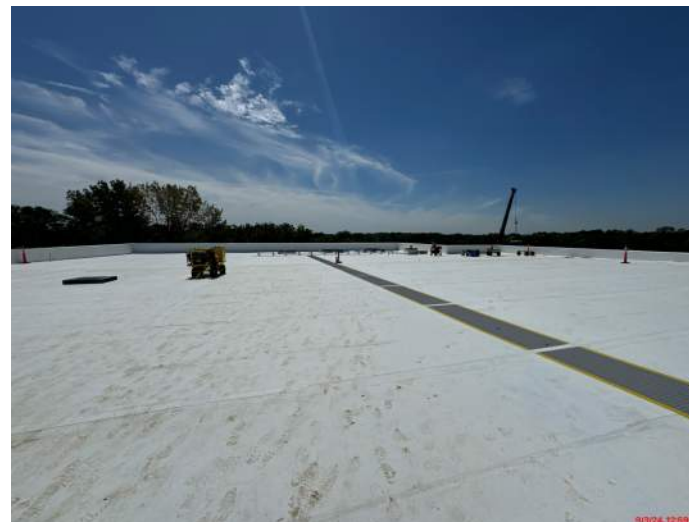
Upper Roofing TPO
