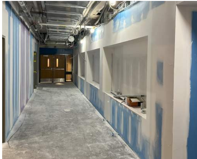
Progress 100's Wing
