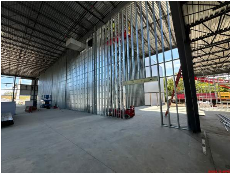
Warehouse Divider Wall
