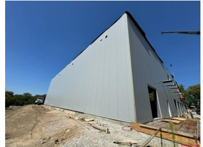
Metal Panels South Wall
