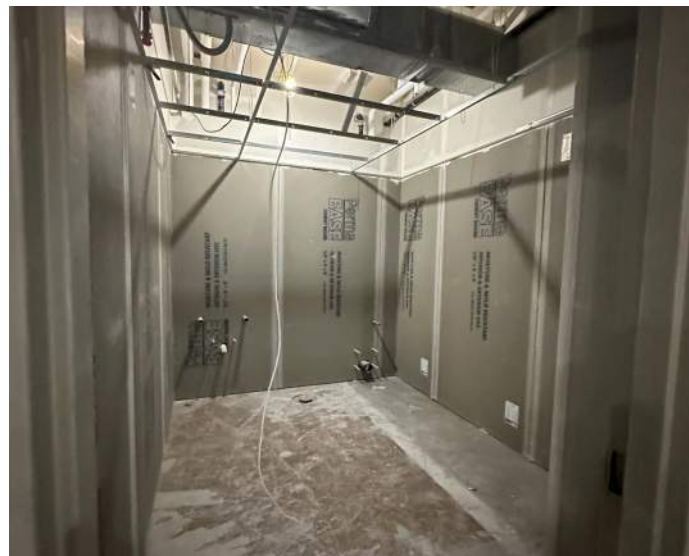
Progress 100's Wing
