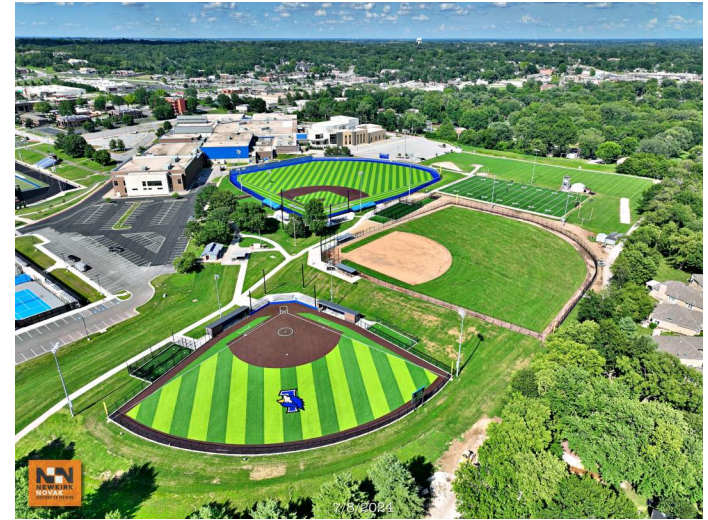
LHS - Overall Site
