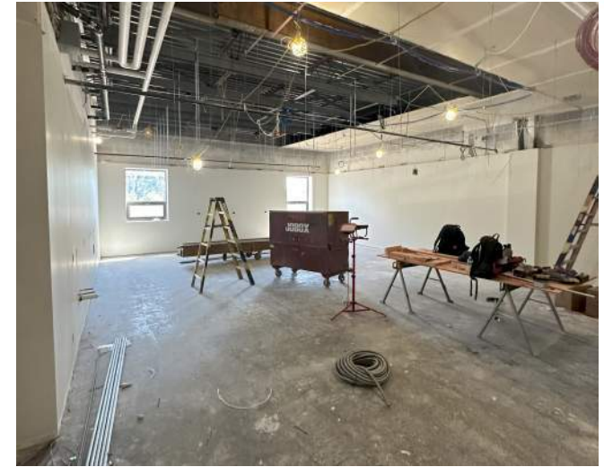
Progress 100's Wing
