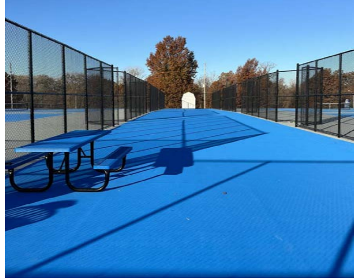
Center Spectator Concourse Looking West
