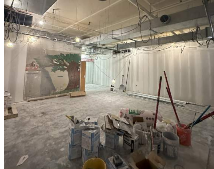
Progress 100's Wing
