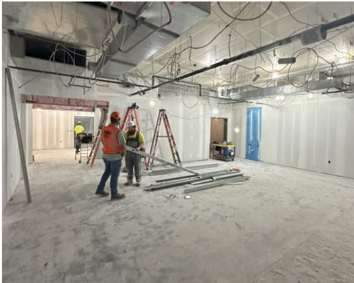
Progress 100's Wing
