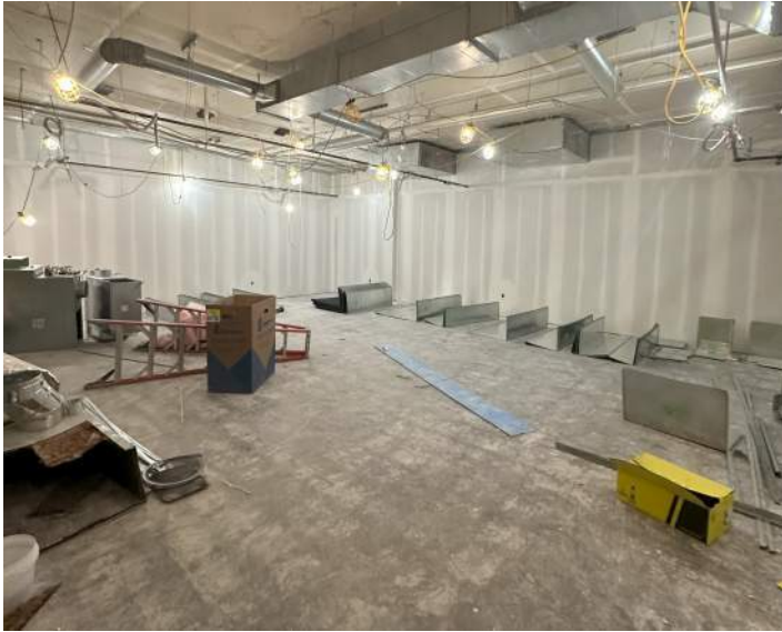
Progress 100's Wing
