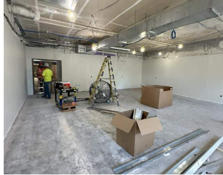
Progress 100's Wing
