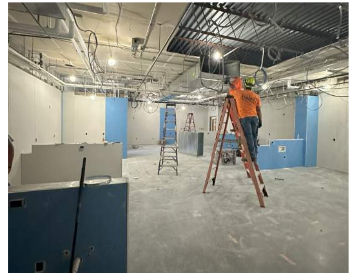
Progress 100's Wing
