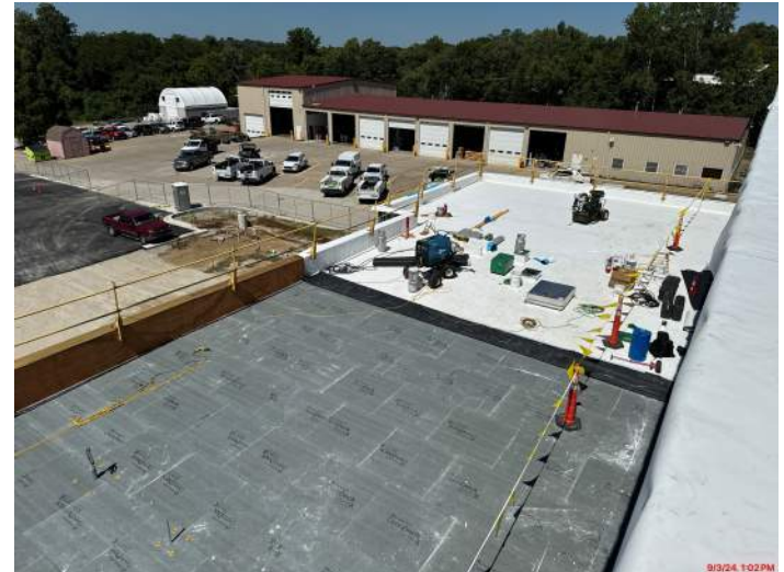
Lower Roofing TPO
