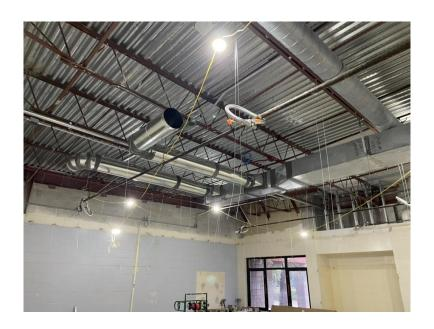
Photo: Additions to existing ductwork for A/C efficiency.
