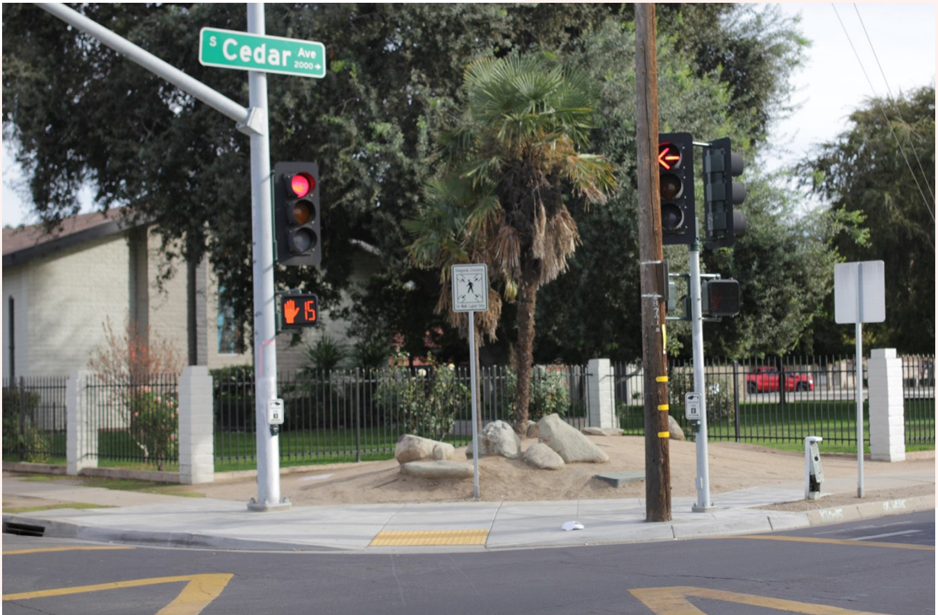
Instructional sign at pedestrian scramble crosswalk, Cedar and Woodward Avenues
