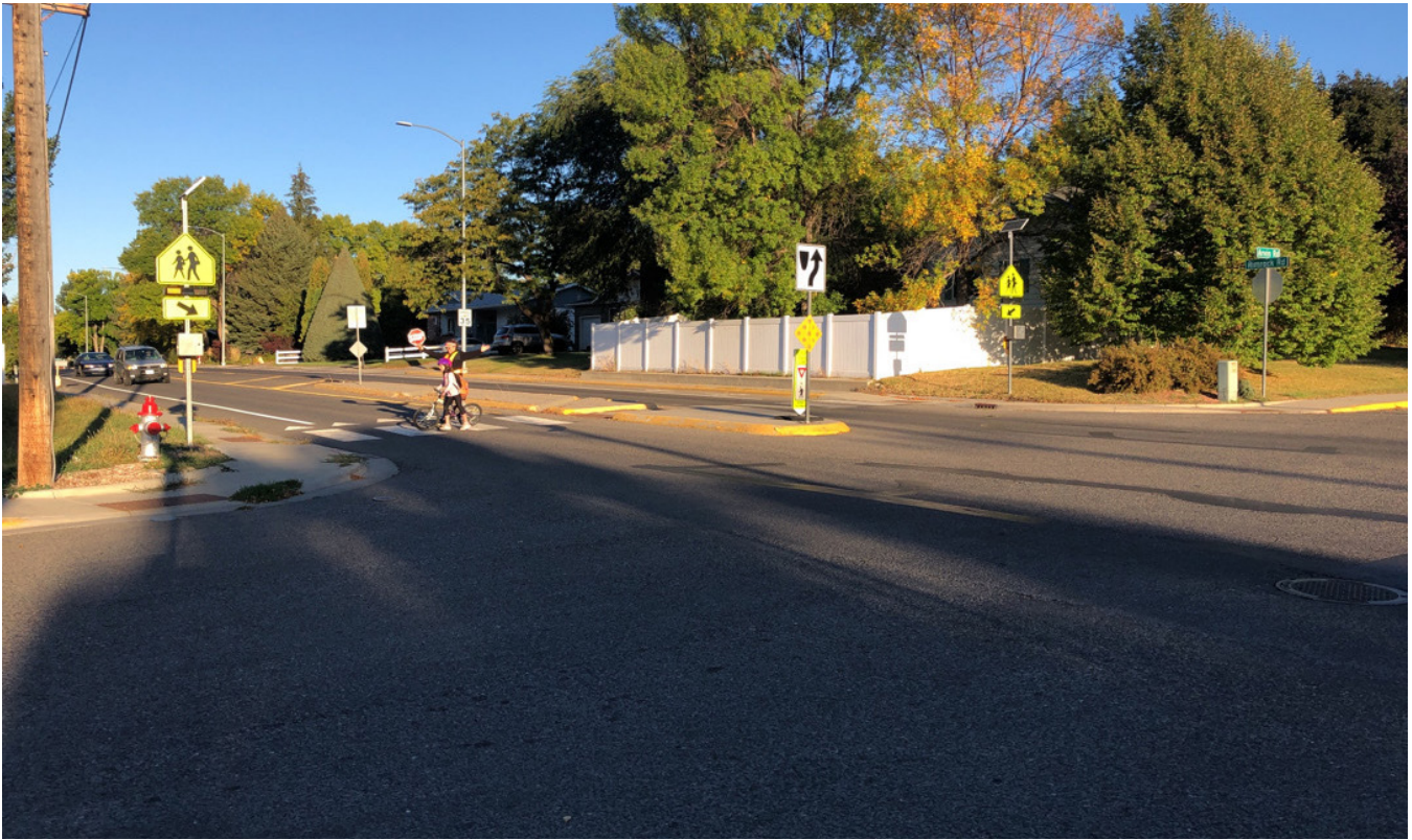
Ample school crossing signage at this intersection in Billings, MT, including in the median refuge, is an example of a gateway treatment
