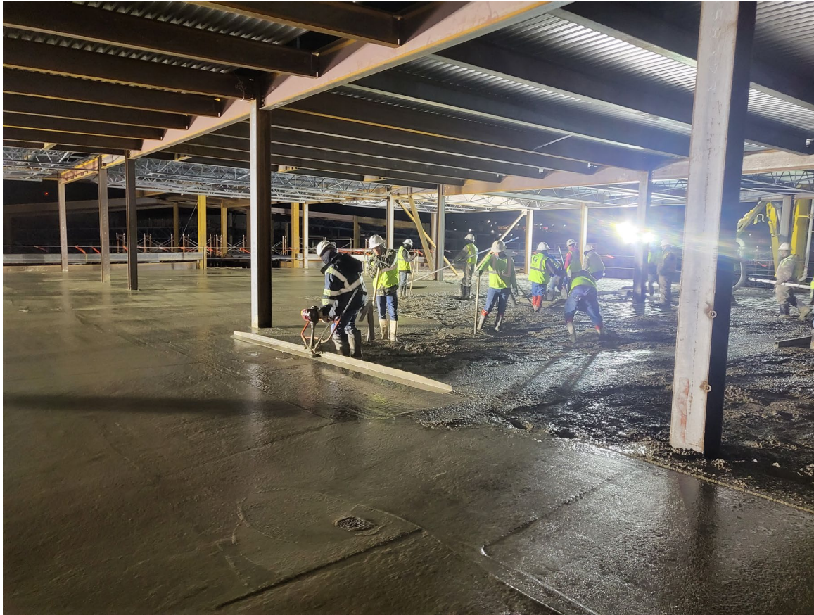
Classroom view when pouring concrete January 12, 2024
