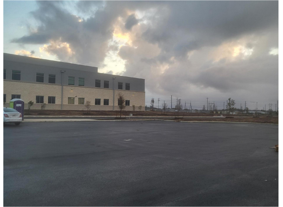
Landscaping Tree Install
