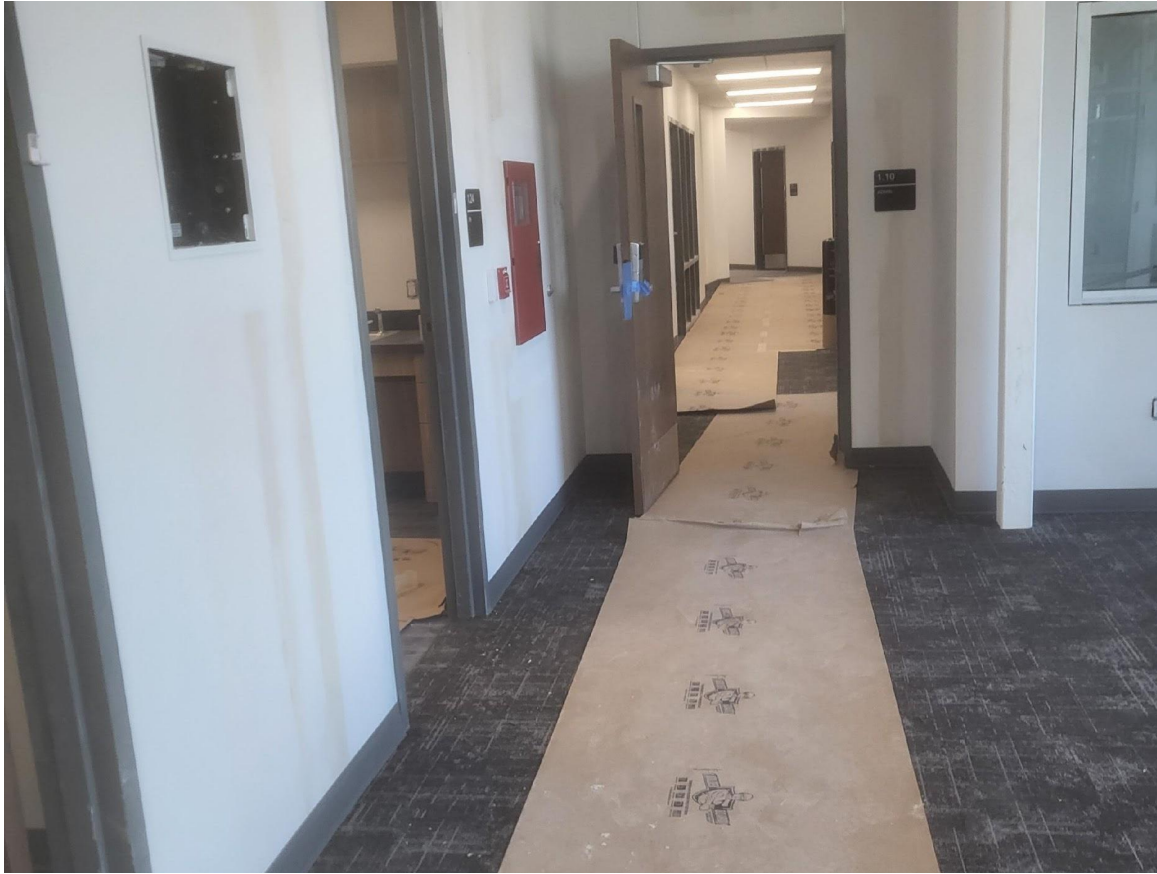
Admin area carpet installed
