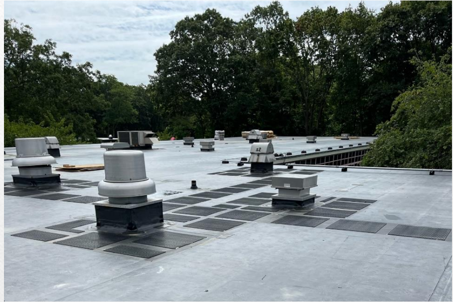
Pictured above is the completed Roof Project at Cherry Avenue – Summer 2023
