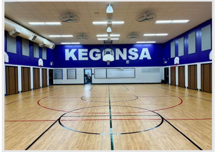
Top Right: a view of the gym / cafeteria following the new floor and striping install, new light fixtures, ceiling, acoustical panels, and paint
