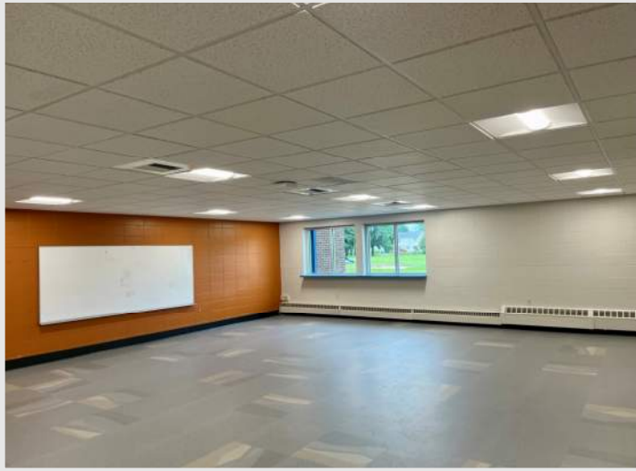
Top Left: a view of the completed finishes in a classroom in the "orange wing" of Kegonsa Elementary
