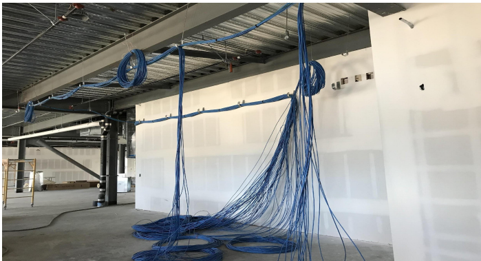
Data infrastructure installation (January 2024)
