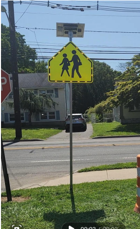
Crosswalk Sign added to Middle School Driveway
