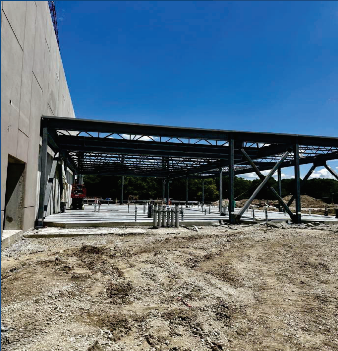
Kitchen Structural Steel Erection
