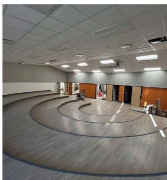
SLP High School Music Renovations – Band Room
