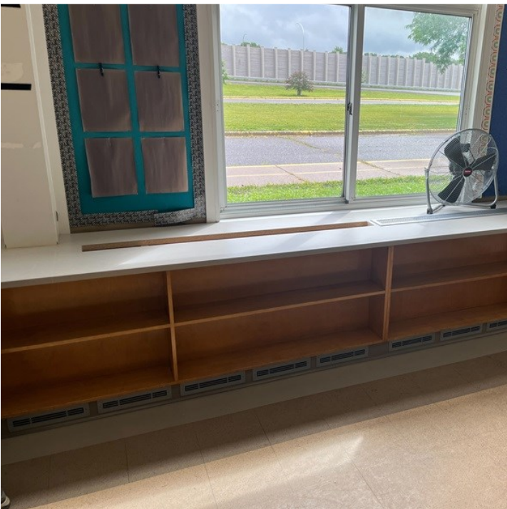
From top left: New boilers and piping; casework modifications for fin-tube radiant heat piping (August 2024)
