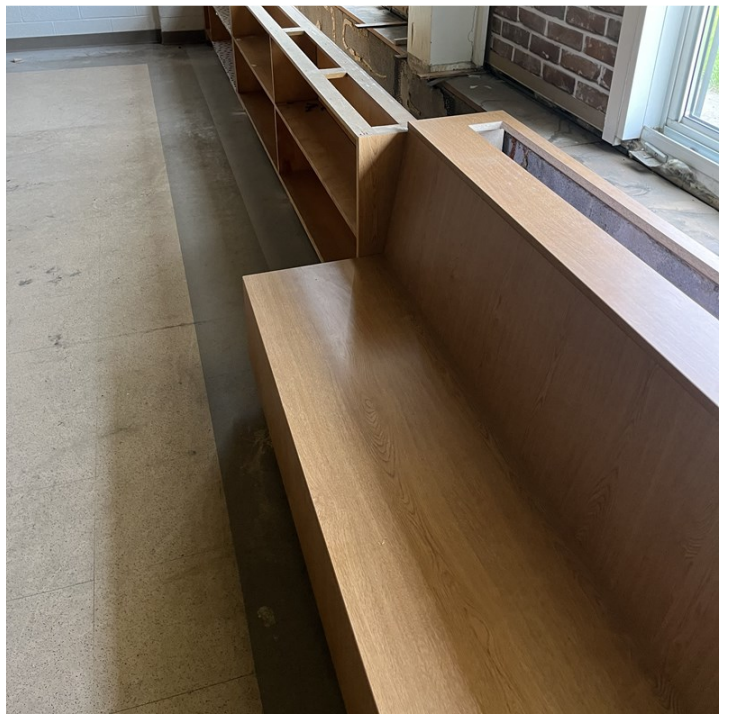
From top left: New boilers and piping; casework modifications for fin-tube radiant heat piping (August 2024)
