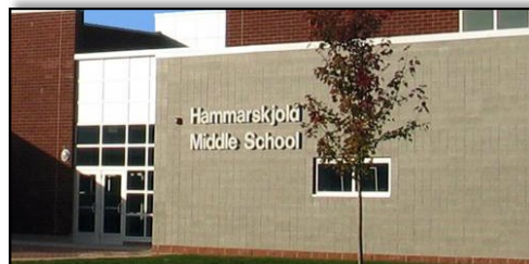
Hammarskjold Upper Elementary School 200 Rues Lane 732-613-6892
