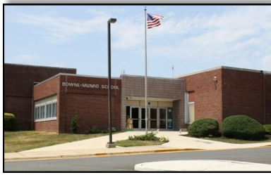
Bowne-Munro Elementary School 120 Main Street 732-613-6810
