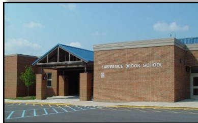
Lawrence Brook Elementary School 48 Sullivan Way 732-613-6872
