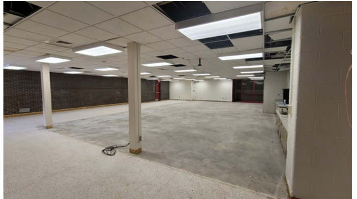
Media Center - During Construction
