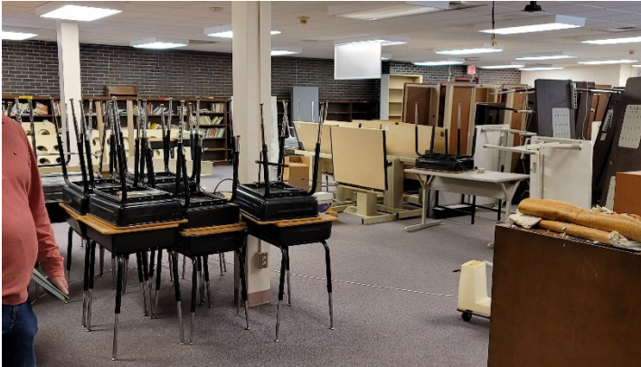
Media Center - Before Construction
