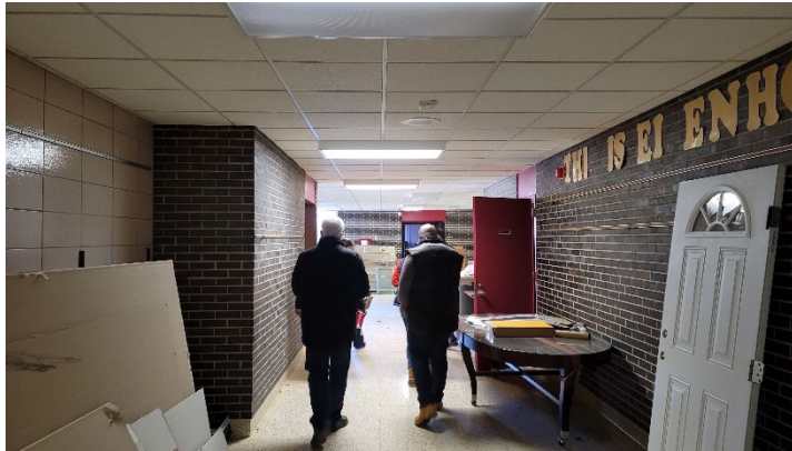
Common Areas - Before Construction
